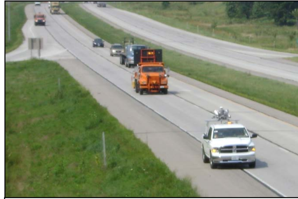
Scanning with Traffic Control
