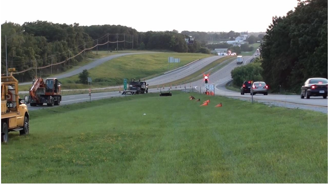
Figure 2.6 I-70 WB at mile marker 131, three-head signal.
