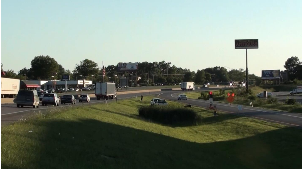
Figure 2.10 I-70 WB at mile marker 125.6.
