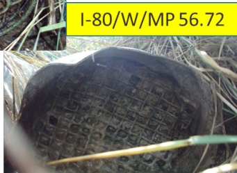
Blocked Outlet with Mesh Gate Screen Opened Outlet without Mesh Gate Screen
