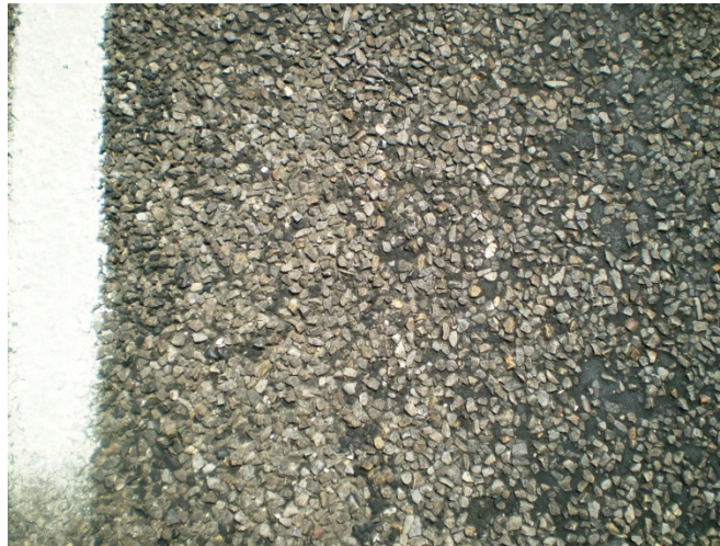
Figure 33. Field Performance under Heavy Traffic—HS A-6.
