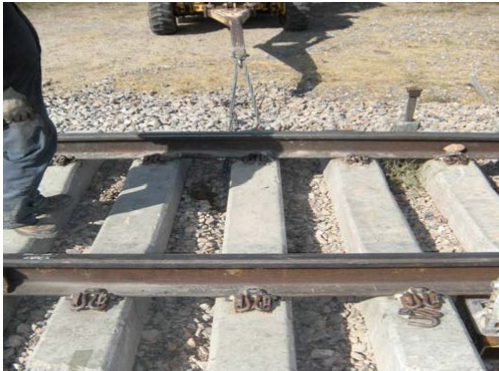
Figure 6. Ballast Being Disturbed and Removed from under the Ties
