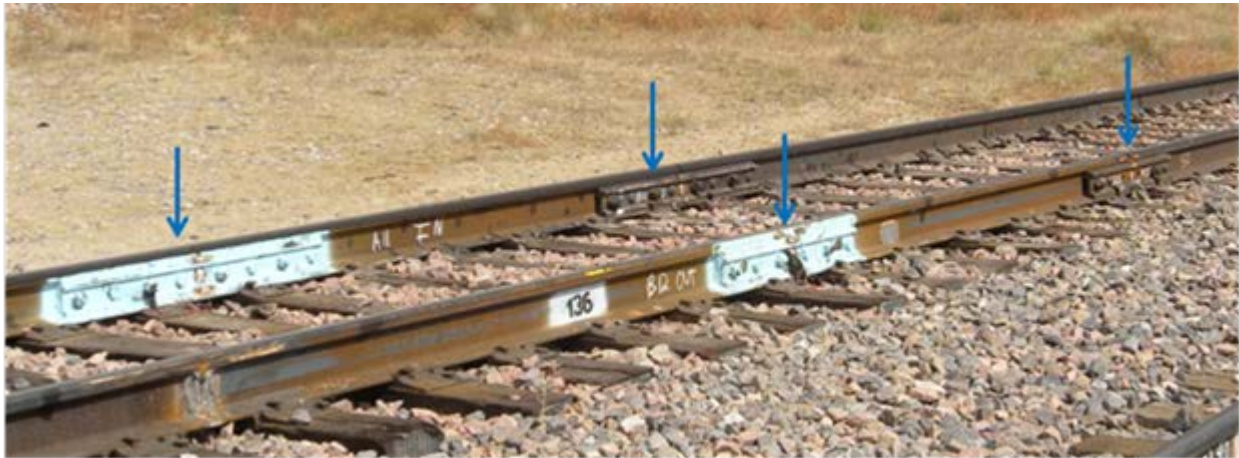
Figure 3. Insulated and Standard Joints installed as Part of the Test
