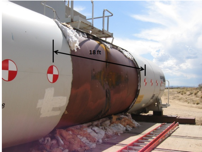
Figure 43. Deformation of Commodity Tank
