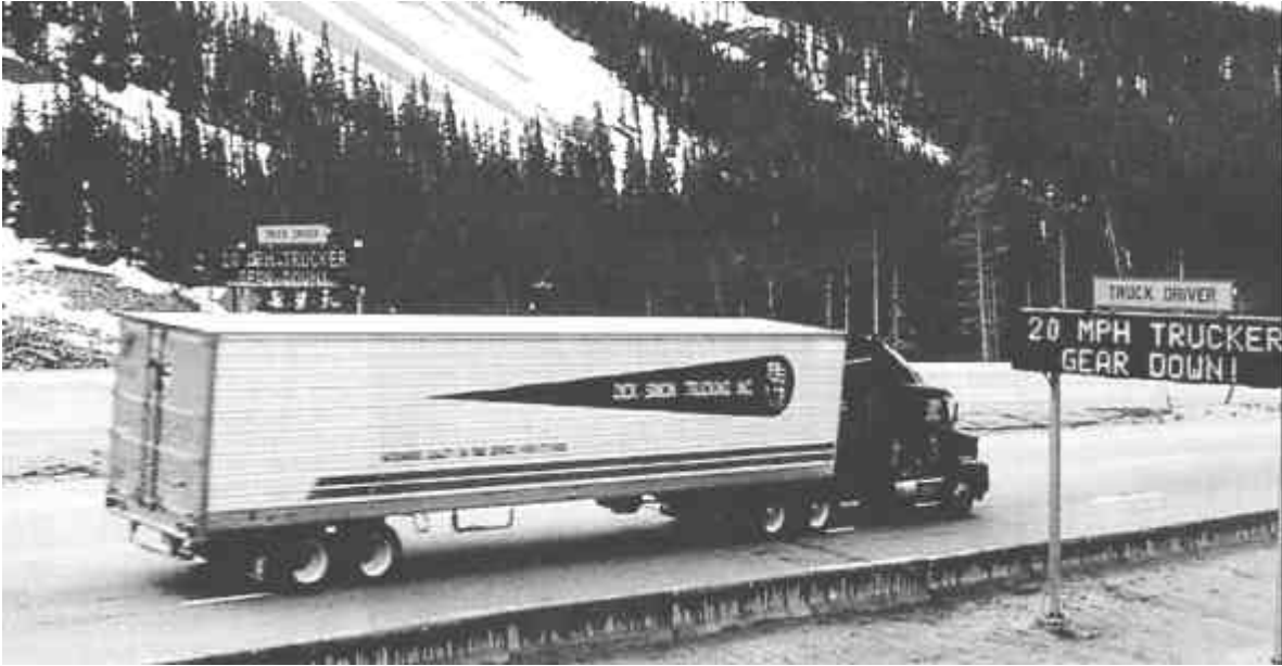
Figure 3-2 Down Grade Warning System installed in Colorado
