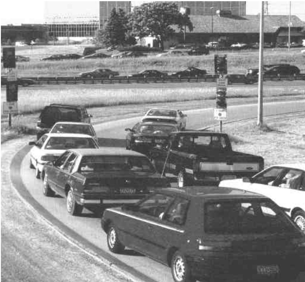
Figure 3-1: Entrance Ramp Meter
