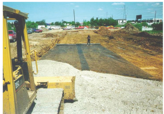
Figure 2.1 Construction procedure for soil-geogrid-aggregate systems.
