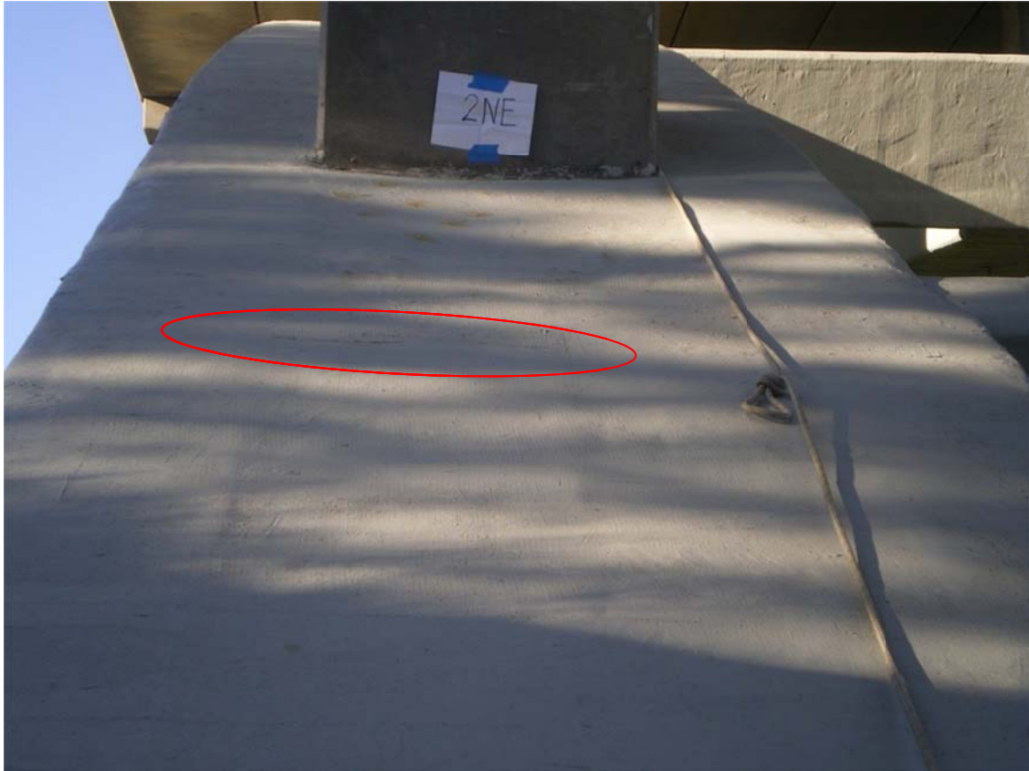
Figure A7. Bay 2NE, Crack enclosed in red oval was identified in 2007
