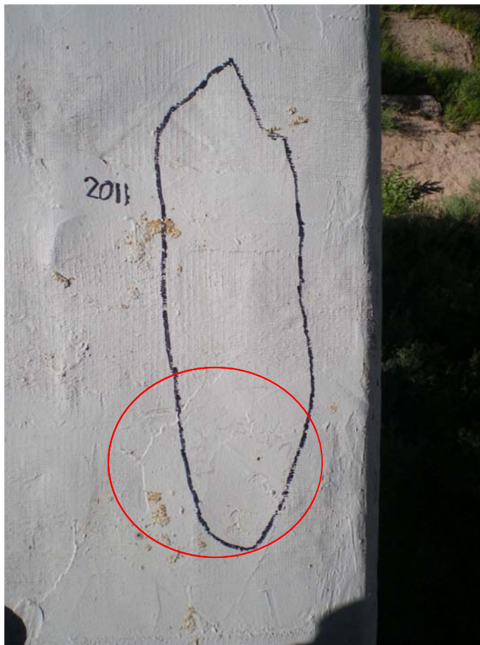
Figure A11. Enclosed in the red circle is 1 of the 2 voids found in 2007
