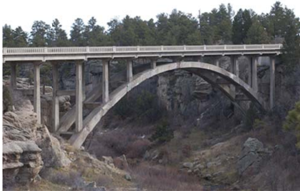
Figure 2.3. Castlewood Canyon Bridge prior to the 2003 repair (Mohseni, CDOT)
