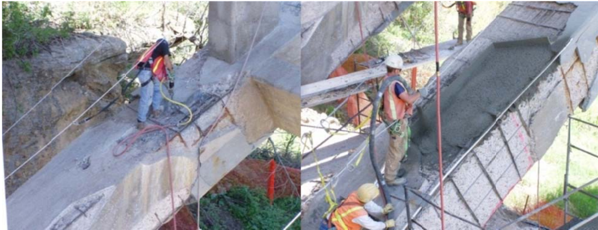
Figure 2.9. Removal of loose concrete using 6.8 kg (15 lbs.) jackhammer and restoring the cross section with shotcrete (Mohseni, CDOT)
