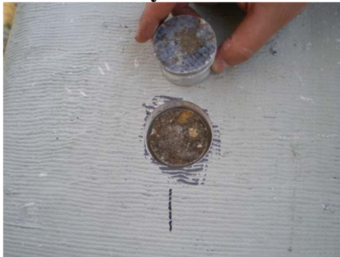
Figure B9. Test No.10, weak bond strength, and test No.11 not available, cored area failed during drilling
