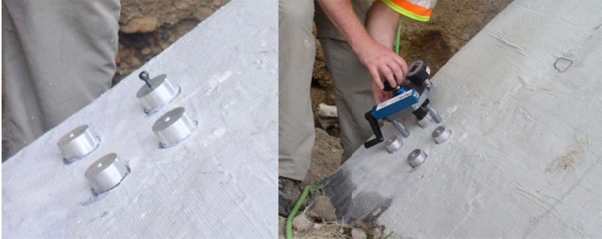
Figure 3.12. Spherical headed bolt threaded into puck and placing the pull-off tester to engage the spherical headed bolt
