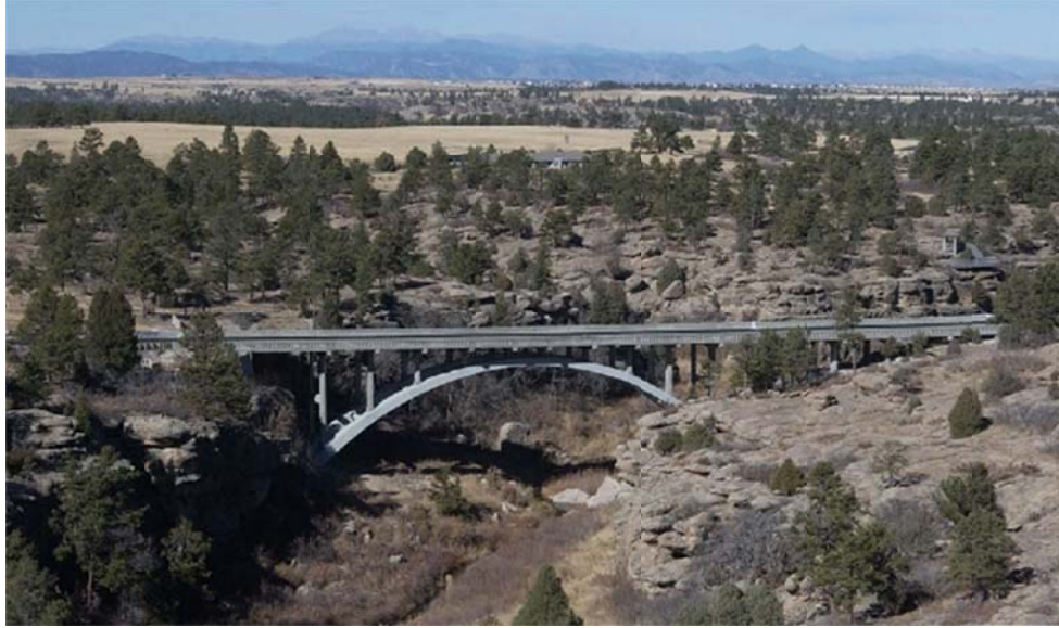
Figure 2.2. Castlewood Canyon Bridge (Mohseni, CDOT)
