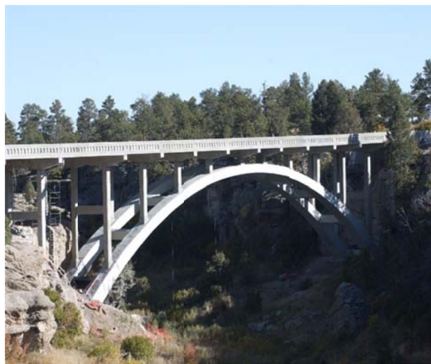
Figure 2.4. Castlewood Canyon Bridge after the 2003 repair (Mohseni, CDOT)
