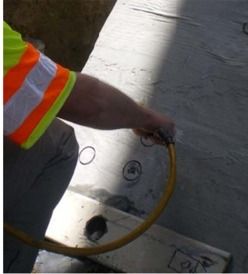
Figure 3.7. Removing water and debris from core cuts
