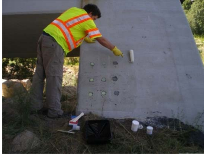
Figure 3.25. Applying a primer coat to the areas for repair
