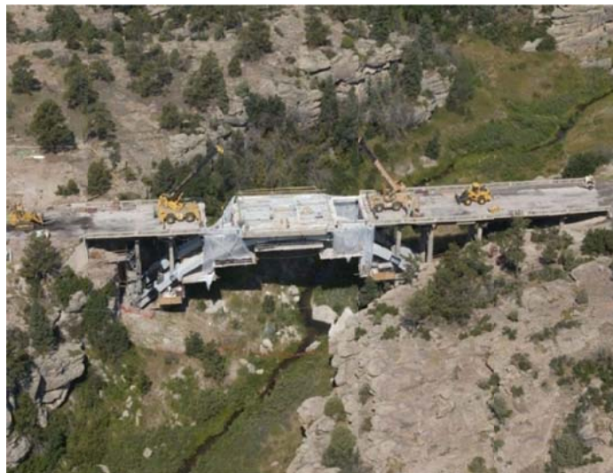
Figure 2.6. Systematically replacing the bridge deck (Mohseni, CDOT)
