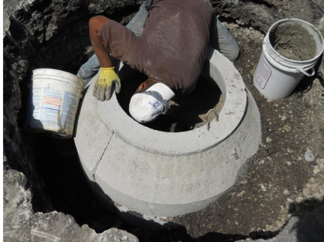
Illustration 2-3. reconstruction of manhole (North Chicago, 2010b)
