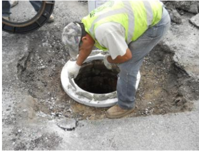
Illustration 2-1. manhole lowering (North Chicago, 2010a)
