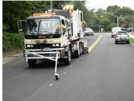
Illustration 2-6. striping paved road (Safety Marking Inc., 2012)
