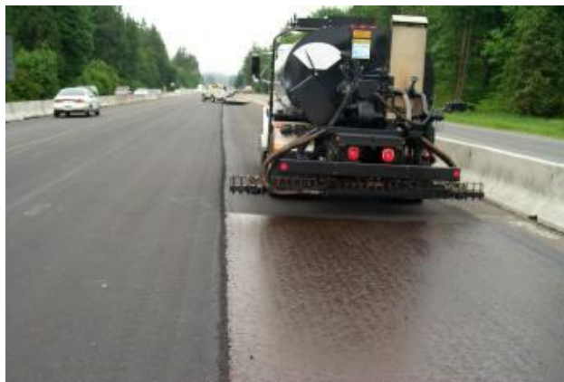
Illustration 2-4. application of tack coat (Pavement Interactive, 2010)
