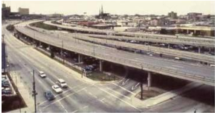
Figure 5: Park East Freeway Before Demolition (Source: The Preservation Institute)
