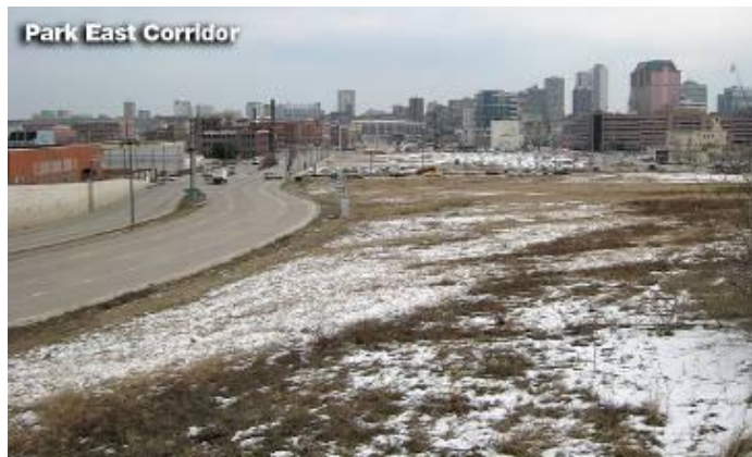
Figure 7: Park East Freeway After Demolition (Source: “Walker Proposes Selling County’s Park East Land to City”, 2009, www.biztimes.com)
