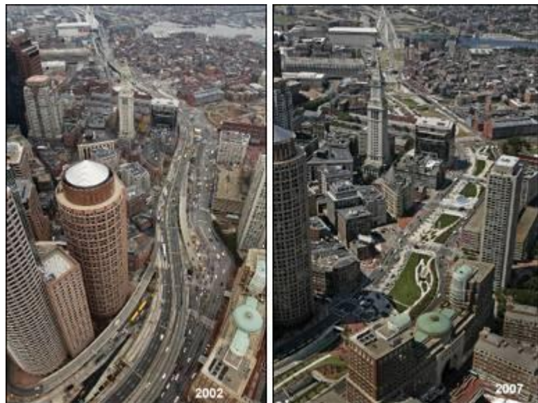
Figure 18: Central Artery Before and After Demolition (Source: Tufts University)
