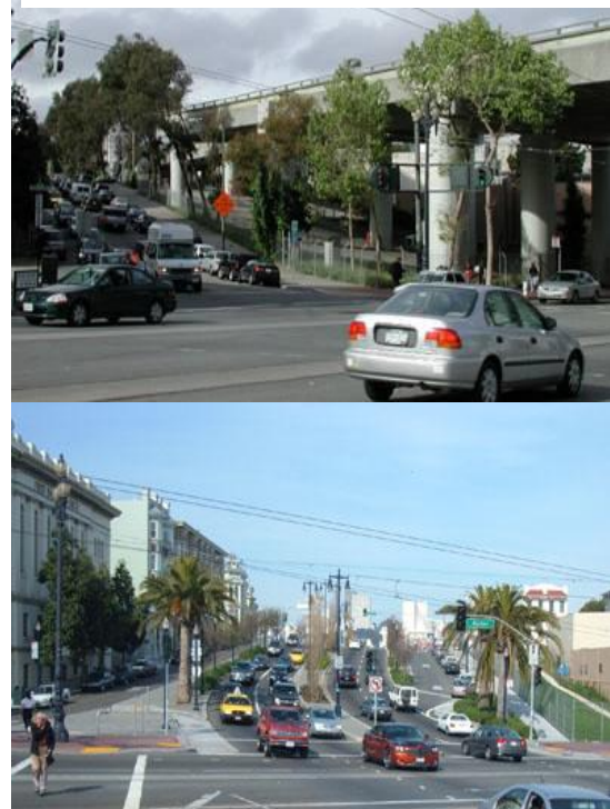
Figure 4: View of Central Freeway Before and After Demolition (Source: The Preservation Institute)
