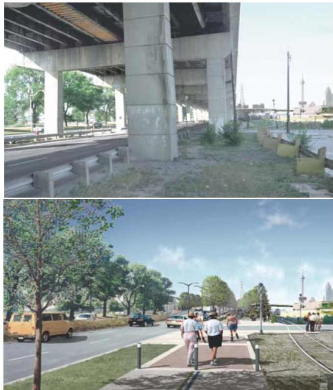
Figure 16: Gardiner Expressway East Before and After Demolition (Source: "Removing Toronto's Elevated Expressway One Piece at a Time: Dismantling the F.G. Gardiner Expressway East")
