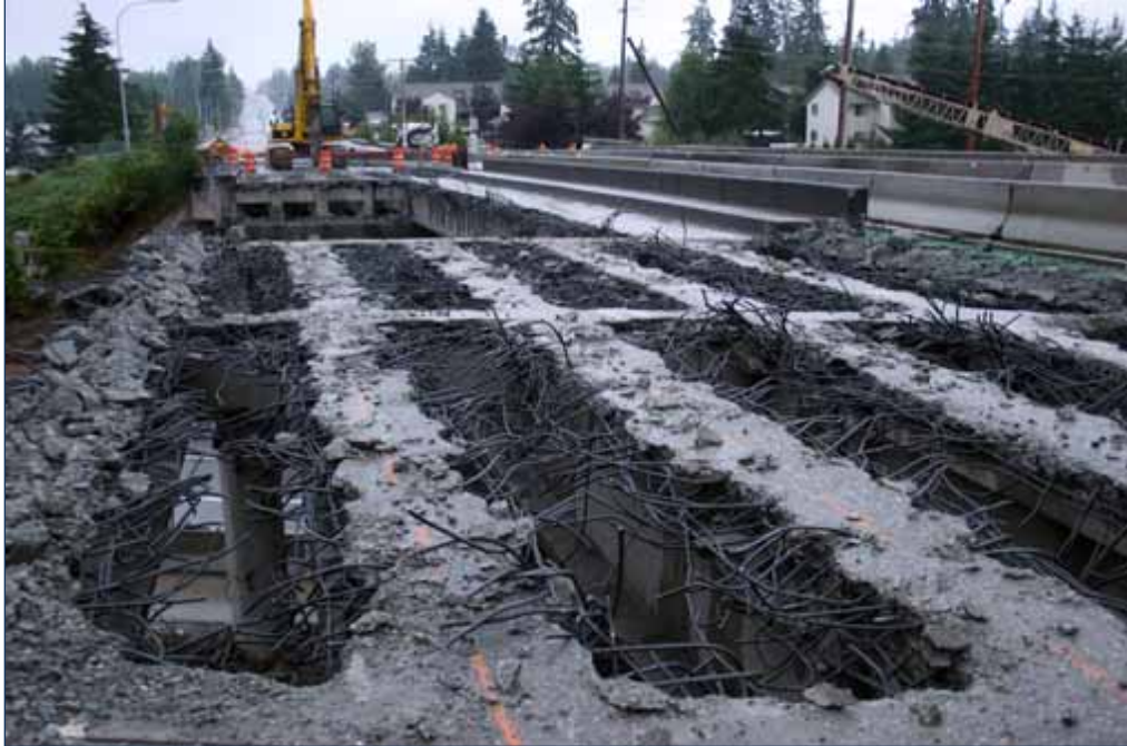
Figure 69. Photo. Existing superstructure with remaining reinforcement after deck removal.
