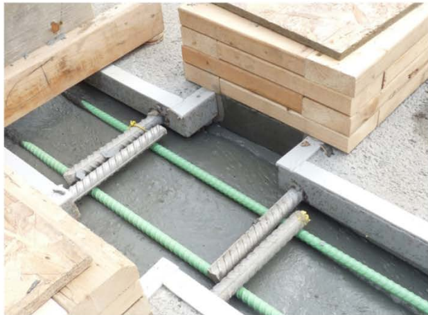
d) Longitudinal joint filled with UHPC
