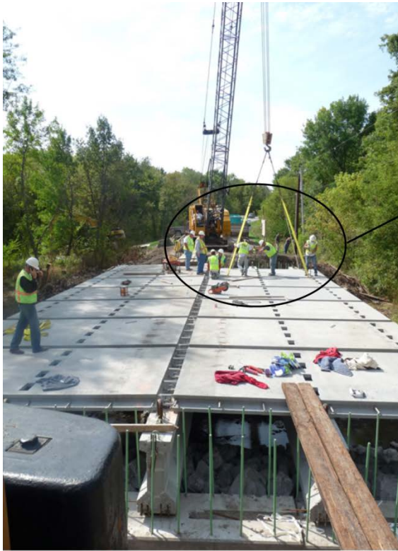
a) Installation of UHPC waffle deck panels
