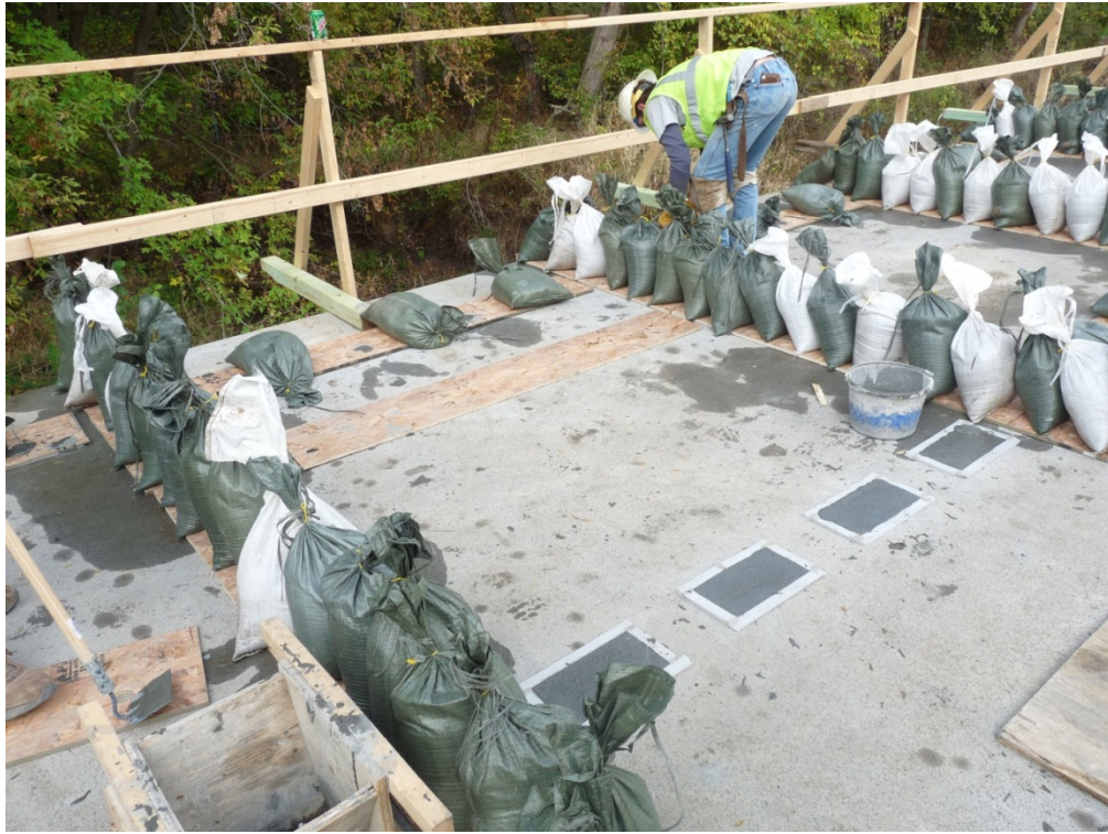
Figure 83. Photo. Finished transverse connections (panel-to-panel connection) covered with plywood.
