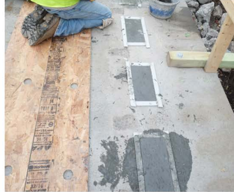
c) Shear pocket with UHPC joint fill
