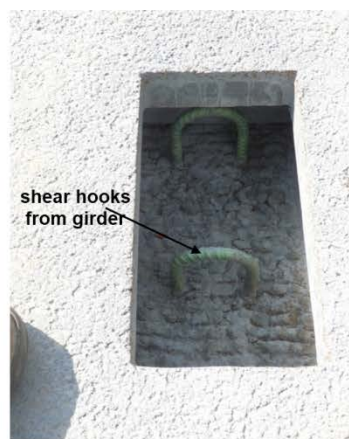
d) Shear pocket ( panel-to-girder connection)
