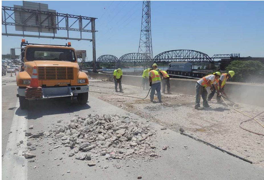
Figure 67. Photo. Jackhammering deck sections prior to removal.
