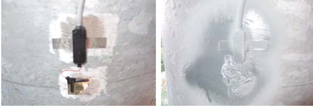
Figure 3.7: Strain gauges mounted on pile
