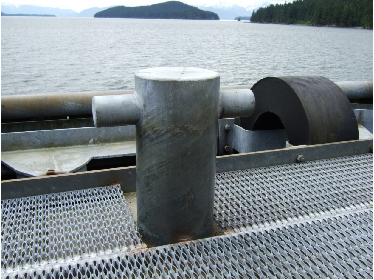
Figure 9: Typical bollard at Auke Bay ferry landing
