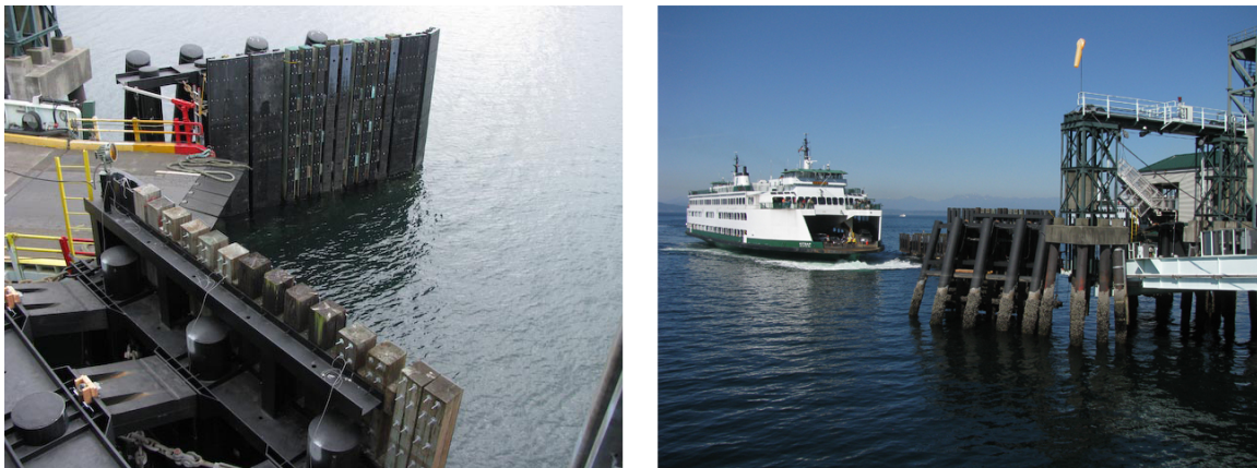
Figure 3.33: Photos of wingwall structure
