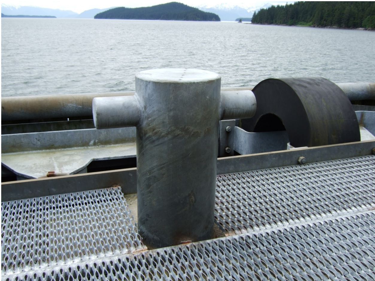
Figure 4.13: Typical bollard at Auke Bay ferry landing
