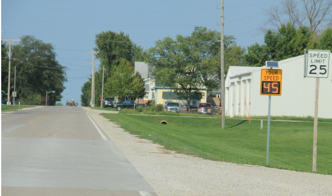
Figure 5-17: DSFS installed at east Rowley community entrance
