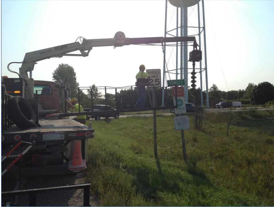
Figure 3-13: Installation of LED speed limit sign
