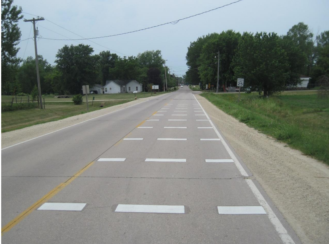
Figure 5-2: Transverse bar treatment at Hazleton east entrance
