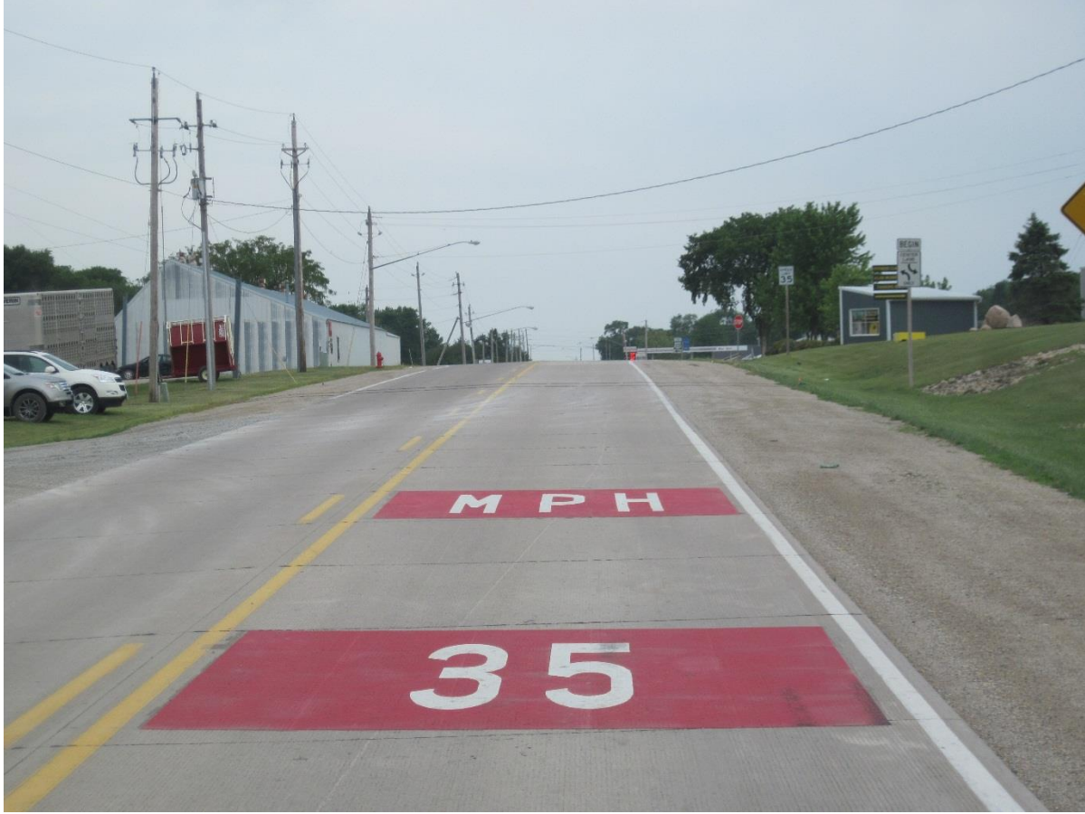
Figure 5-4: Colored entrance treatment for Jesup east community entrance
