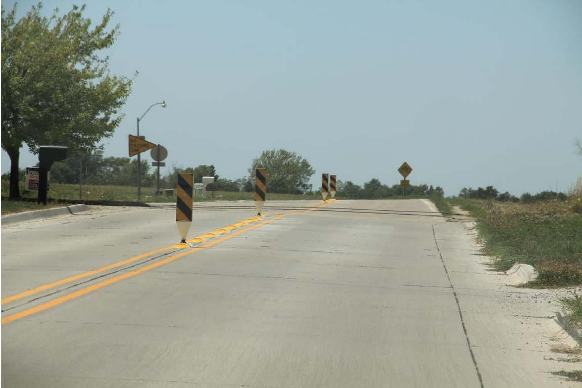
Figure 5-13: Mountable curbing installed at west St. Charles community entrance
