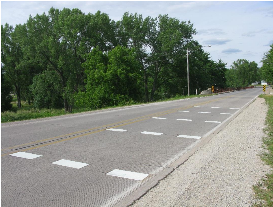
Figure 5-10: Close-up of transverse treatment at south Quasqueton entrance
