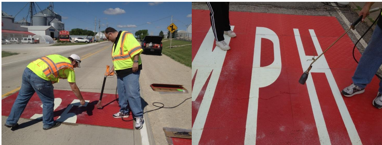
Figure 3-8: Installation of colored entrance treatment
