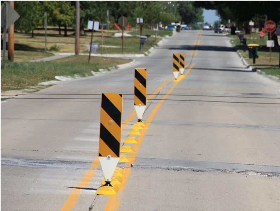
Figure 5-14: Mountable curbing at south entrance to St. Charles
