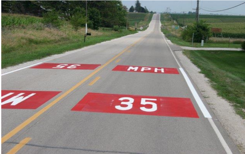
Figure 3-5: European-style traffic-calming treatment used in Dexter, Iowa
