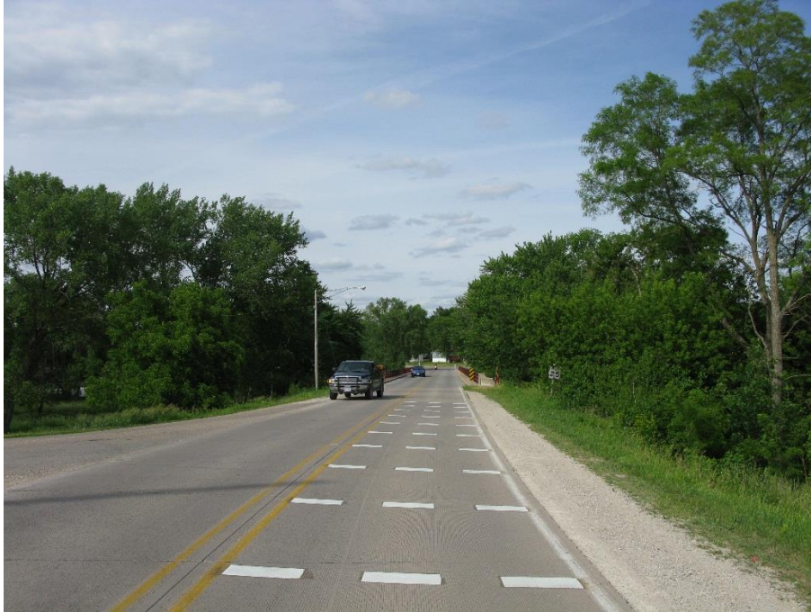
Figure 5-11: Transverse bar treatment at south Quasqueton entrance
