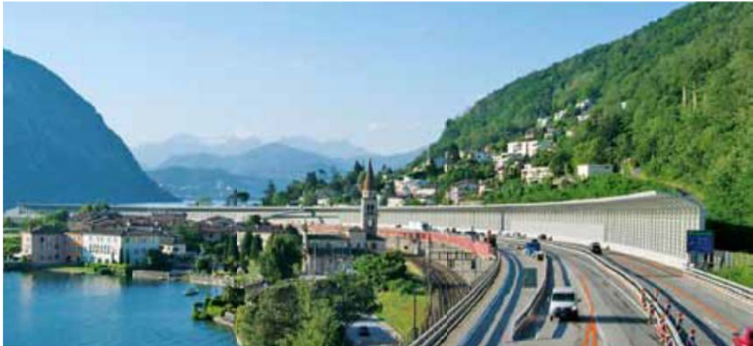
Figure 2. Example of noise barrier with gallery-style top
