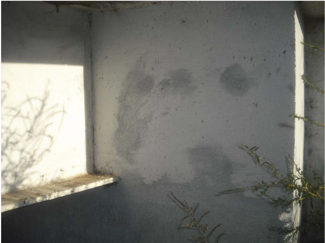
Figure 6: South Abutment of NB Bridge with SCC
