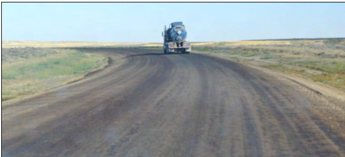
Figure 4.37 Road surface of limestone crushed base treated with lignin and magnesium chloride on uphill, curved segment D of Sweetwater County's Crooks Gap Road in August 2011, three weeks after application of dust suppressant.
