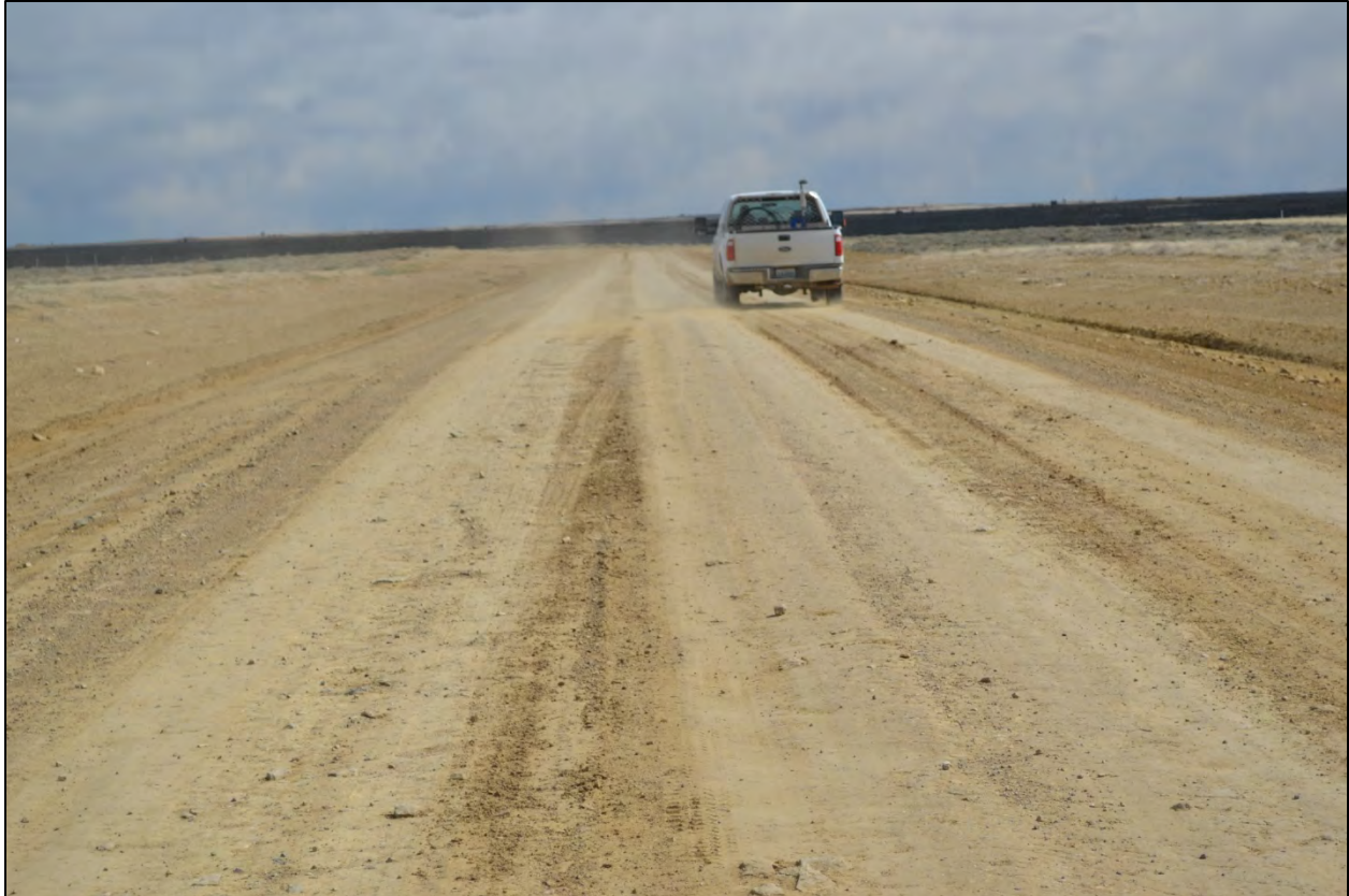
Figure 3.13 Crooks Gap Road north of the test sections showing the surfacing material typical of that which was blended with RAP or CTB on the Sweetwater County test sections.
