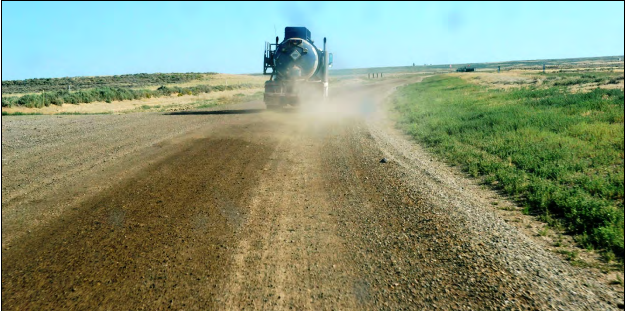
Figure 4.42 Road surface with good crust made of reclaimed cement-treated base treated with polymer and magnesium chloride on segment G of Sweetwater County's Crooks Gap Road in August 2011, three weeks after application of dust suppressant.
