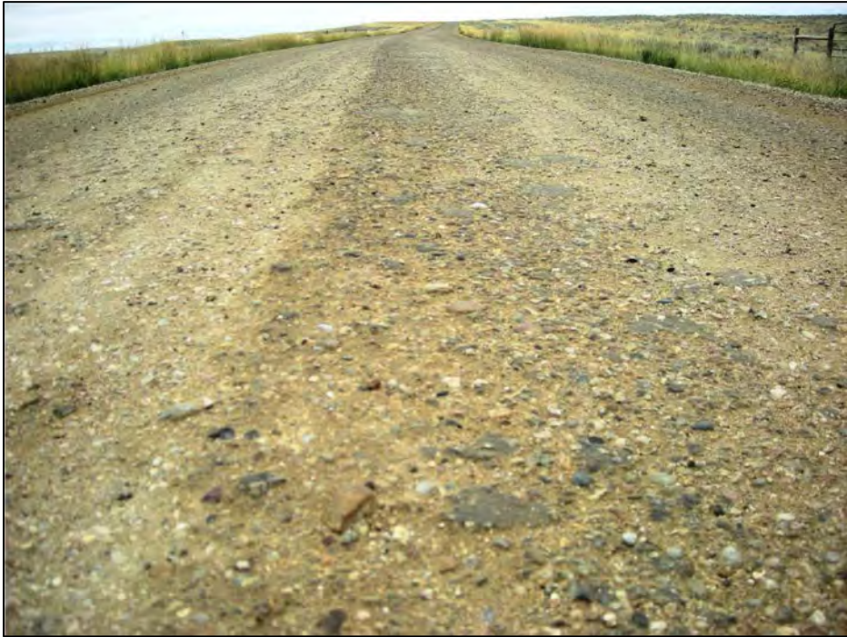
Figure 4.23 Road surface on Johnson County's Schoonover Road, segment S0 with aggregate and calcium chloride in September 2008, two months after calcium chloride application.
