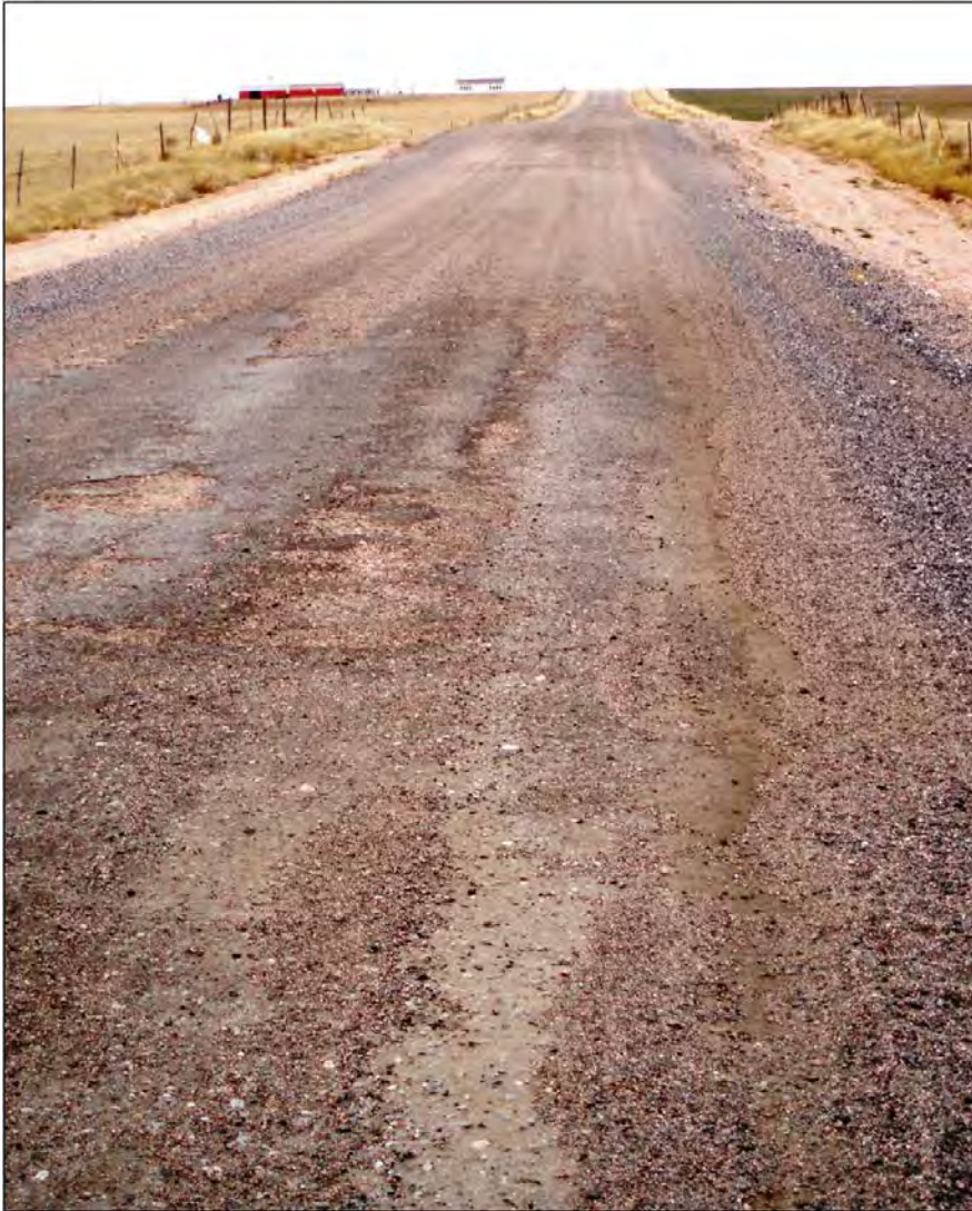
Figure 4.16 Variable densification under traffic due to incomplete blending and segregation of RAP and aggregate on Laramie County's Pry Road in November 2008, six months after initial compaction and three months after re-working.
