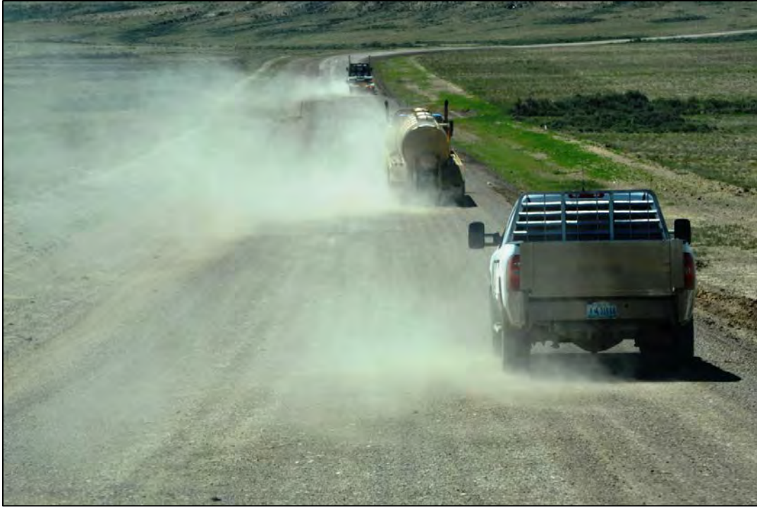
Figure 4.40 Dust from road surfaced with coarser reclaimed cement-treated base on segment E of Sweetwater County's Crooks Gap Road in June 2011 before application of dust suppressants.
