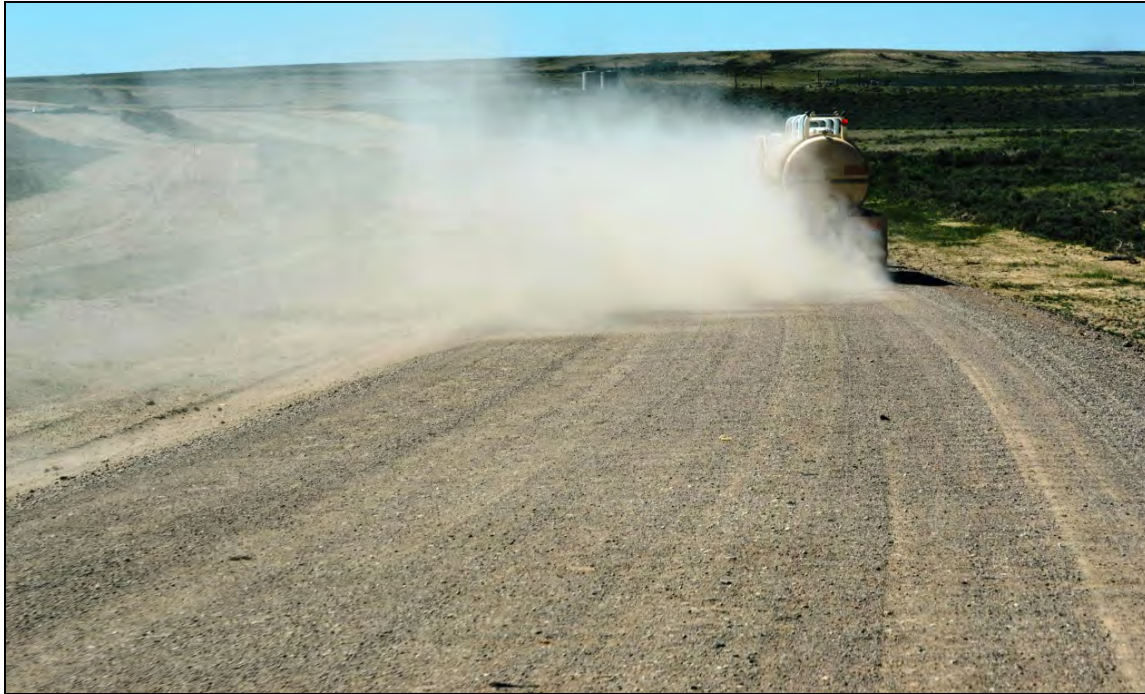
Figure 4.39 Dust from road surfaced with finer reclaimed cement-treated base on segment G of Sweetwater County's Crooks Gap Road in June 2011 before application of dust suppressant.
