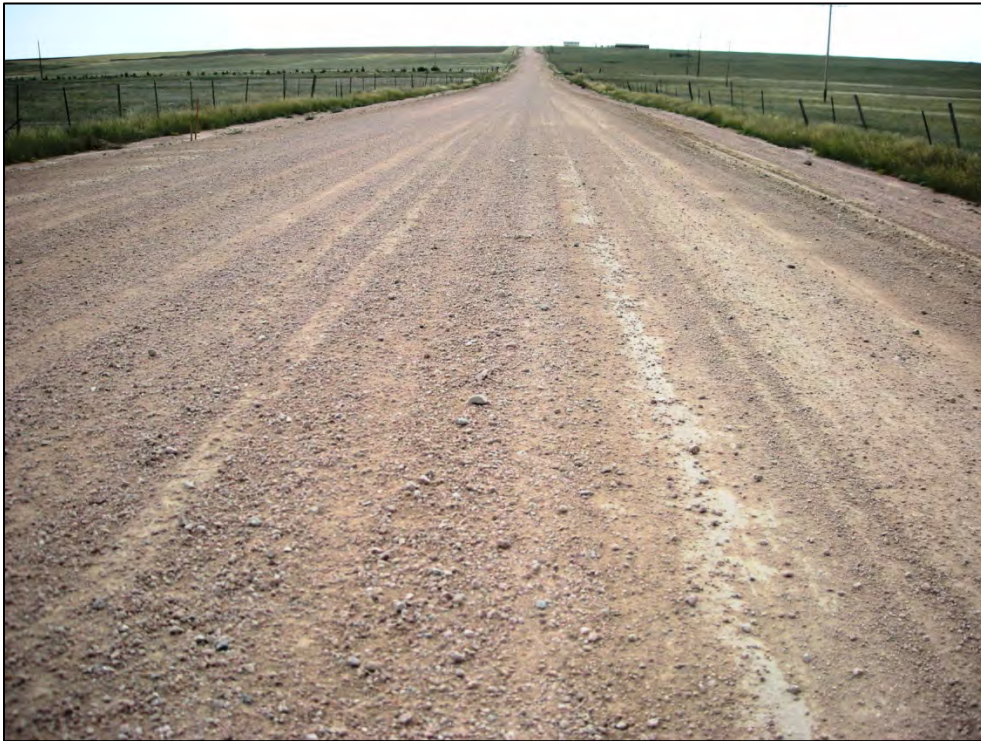
Figure 4.18 Aggregate only forming a good driving surface on Laramie County's Atlas Road in September 2008, four months after shaping.
