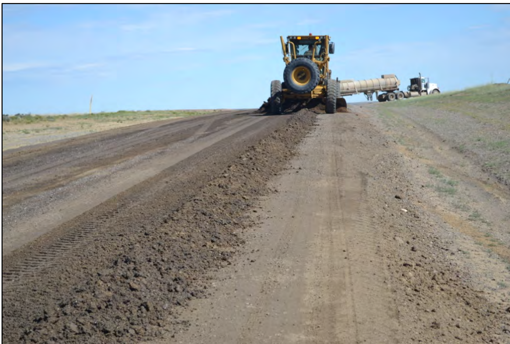
Figure 3.36 Shaping dampened RAP and aggregate blend in preparation for placement of dust suppressants on Sweetwater County's Crooks Gap Road, July 2011.
