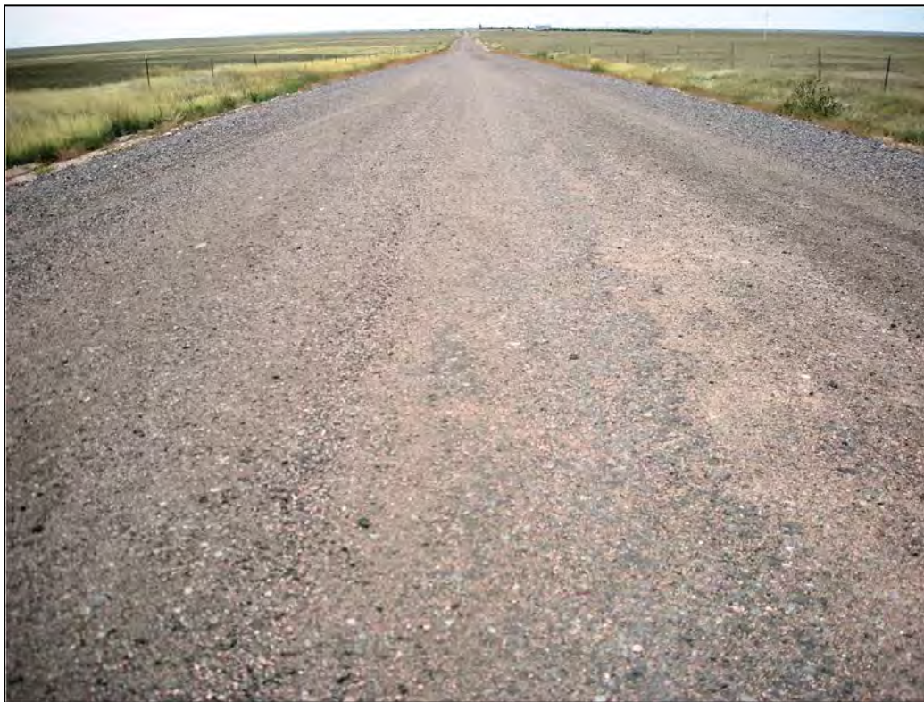
Figure 4.15 Good, tight surface on Laramie County's Atlas Road in October 2008, five months after initial application and two months after re-blending with motor grader.
