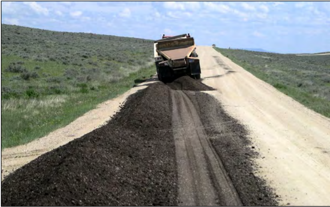
Figure 3.22 Placing RAP and aggregate blend on Johnson County's Schoonover Road, June 2008.
