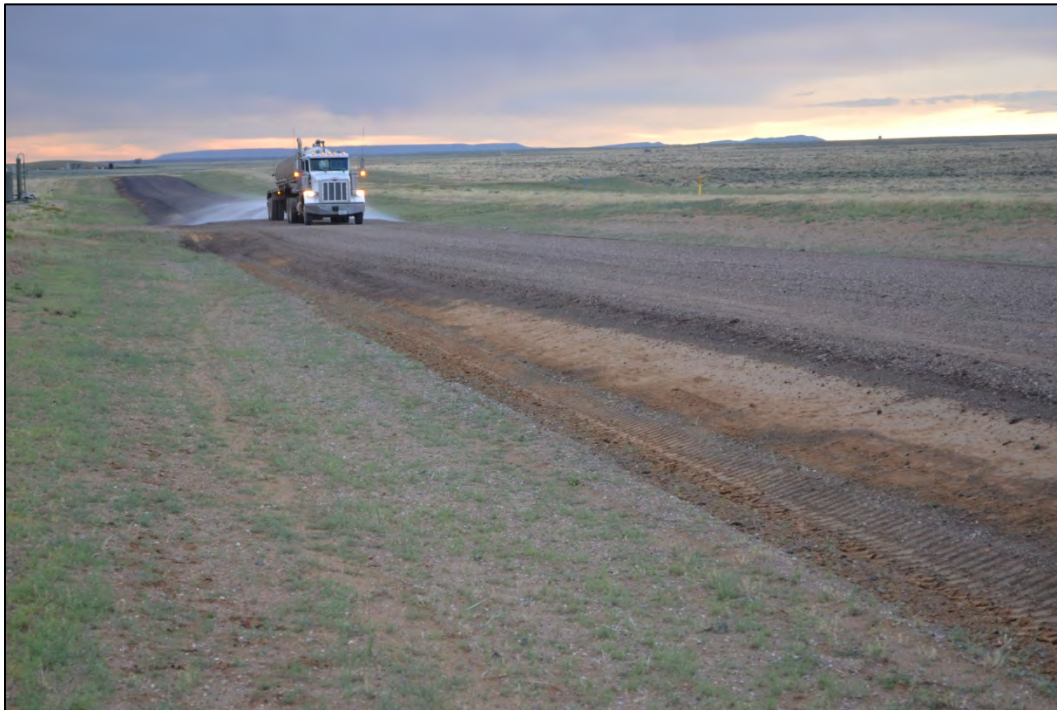
Figure 3.34 Pre-wetting RAP and aggregate blend at dawn prior to application of dust suppressants on Sweetwater County's Crooks Gap Road, July 2011.
