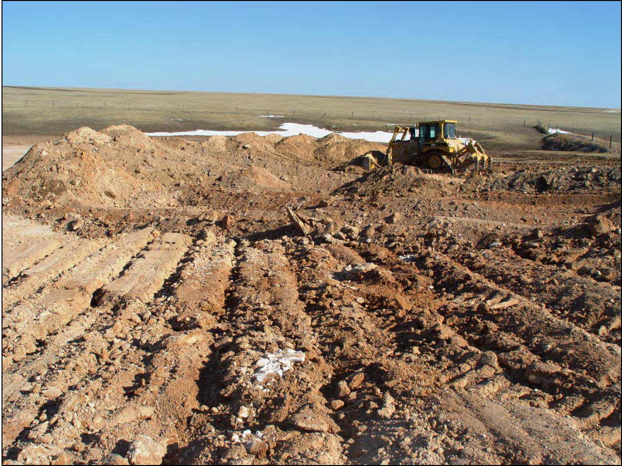
Figure 3.12 Blending of aggregate at Laramie County scoria pit near Atlas Road.
