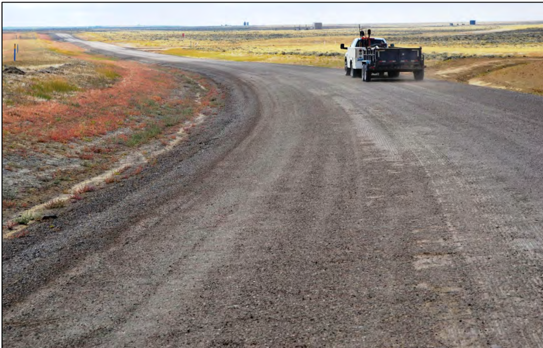
Figure 4.50 Road surface made with RAP blended with existing aggregate and treated with magnesium chloride on segment N of Sweetwater County's Crooks Gap Road in September 2011, eight weeks after application of dust suppressant.
