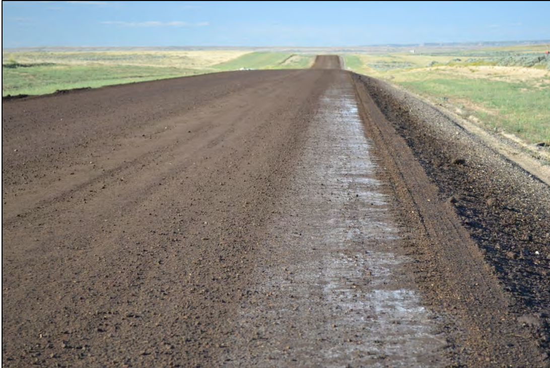
Figure 3.39 Magnesium chloride almost completely absorbed into the RAP and aggregate blend on Sweetwater County's Crooks Gap Road, July 2011.
