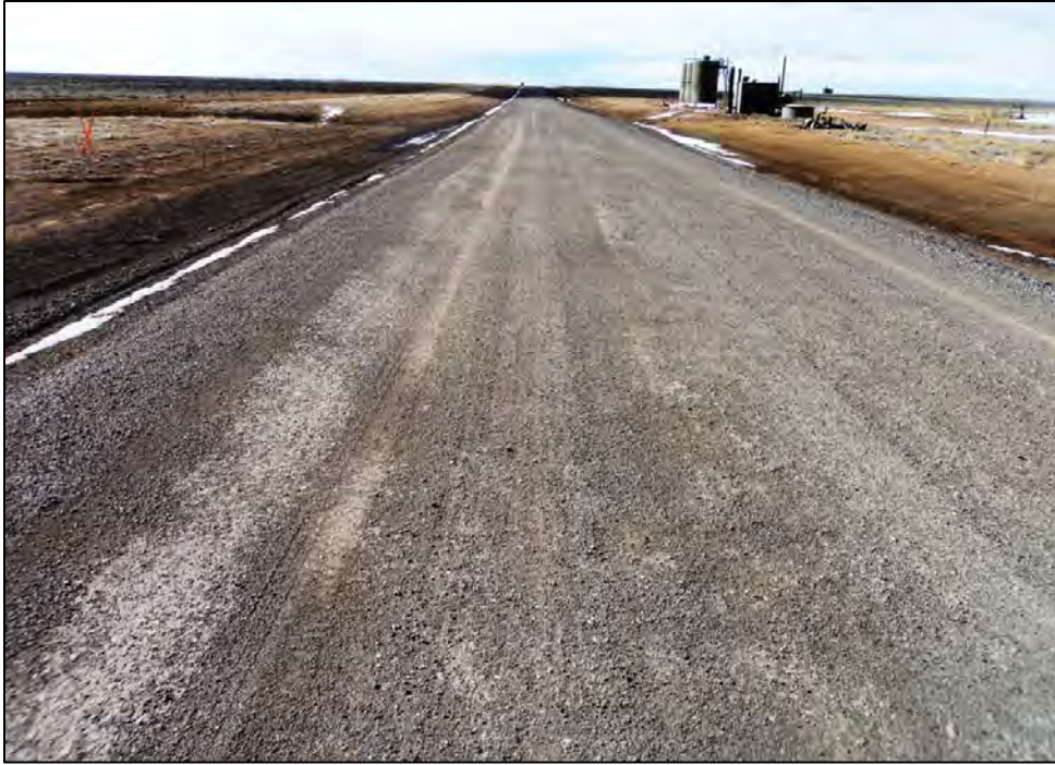
Figure 4.44 Road surface made from RAP blended with existing aggregate on segment M of Sweetwater County's Crooks Gap Road in March 2011, before the application of dust suppressants.
