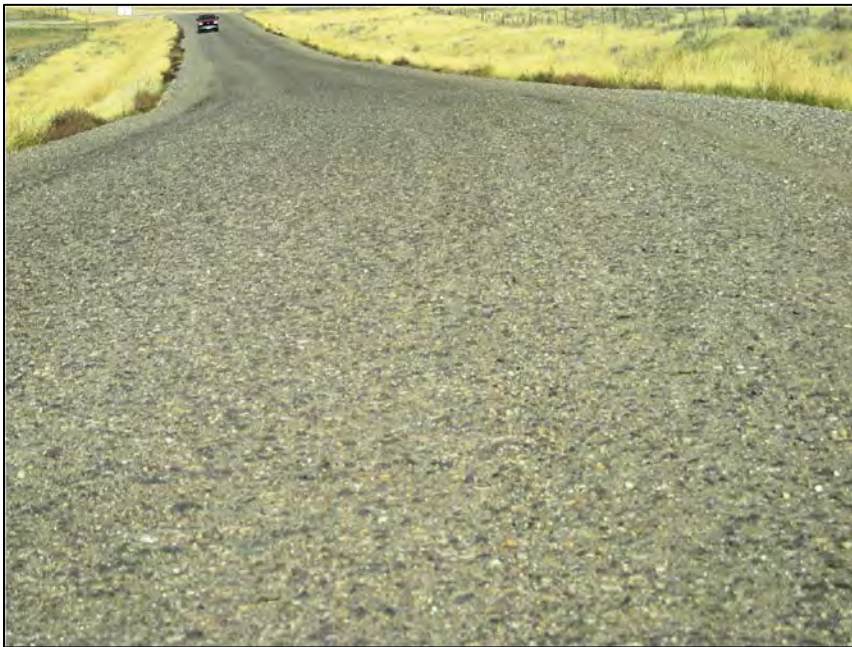
Figure 4.25 Road surface on Johnson County's Schoonover Road, segment S2 with RAP but no calcium chloride in October 2008, four months after RAP placement.
