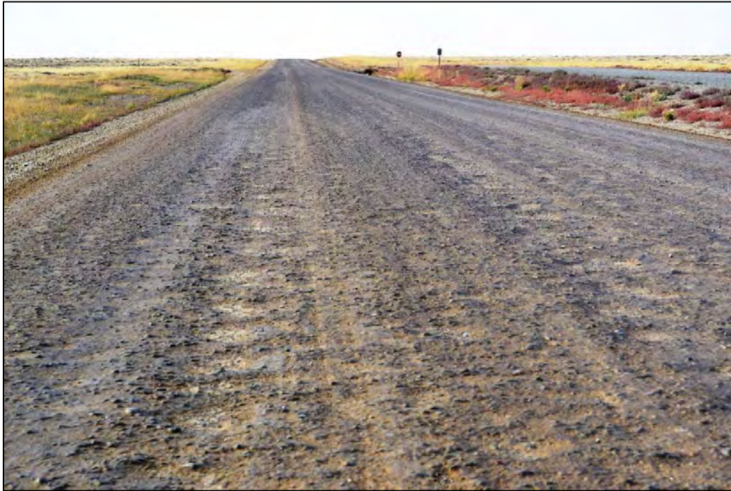
Figure 4.33 Road surface made of limestone crushed base treated with magnesium chloride on Sweetwater County's Crooks Gap Road showing small scale roughness.
