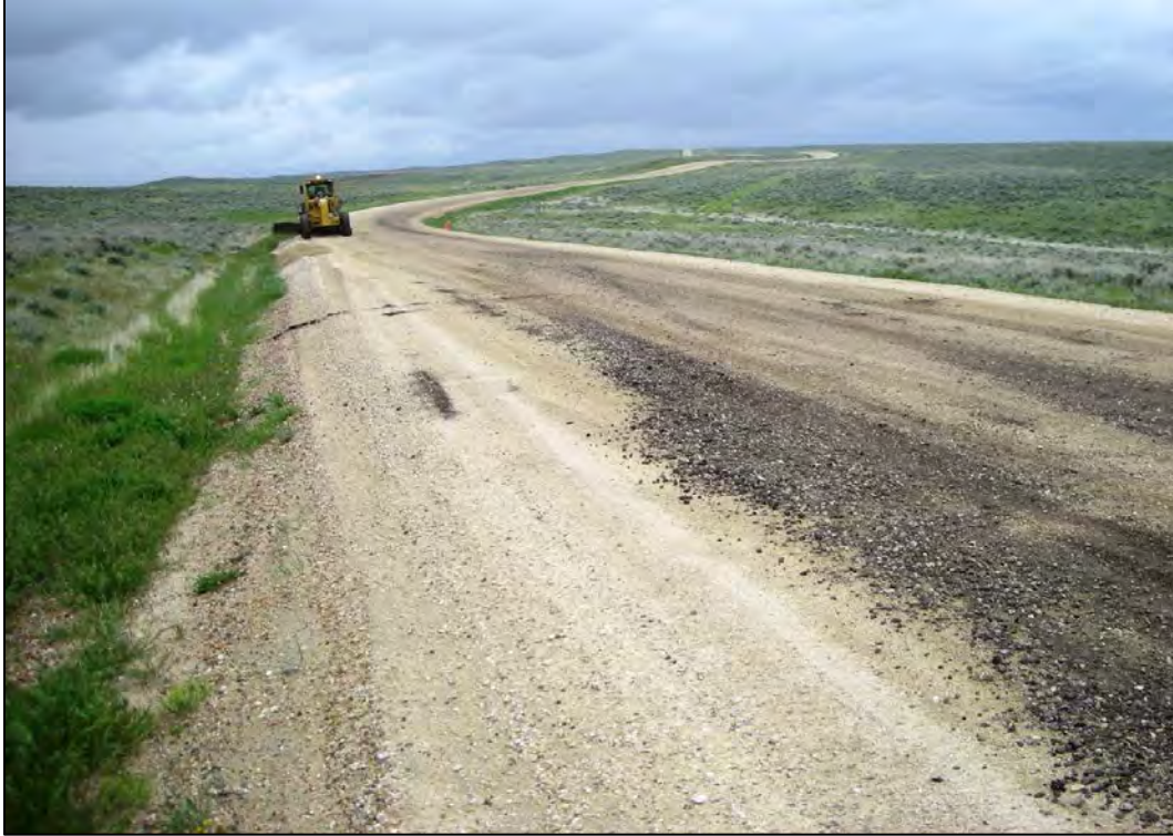
Figure 3.21 Initial shaping of Johnson County's Schoonover Road prior to placement of the blended RAP and aggregate, June 2008.
