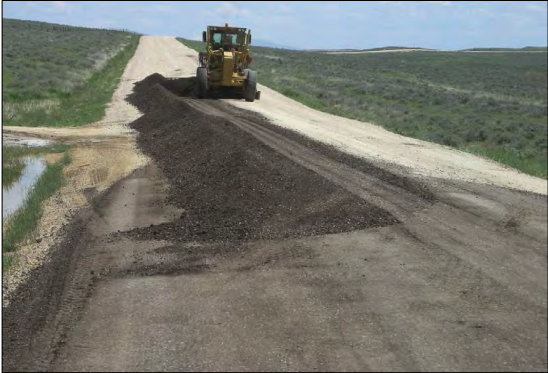
Figure 3.23 Shaping RAP and aggregate blend on Johnson County’s Schoonover Road, June 2008.
