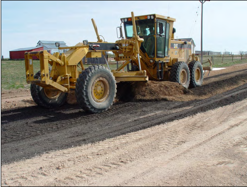
Figure 3.18 Blending RAP and existing, scarified aggregate on Laramie County's Atlas Road.
