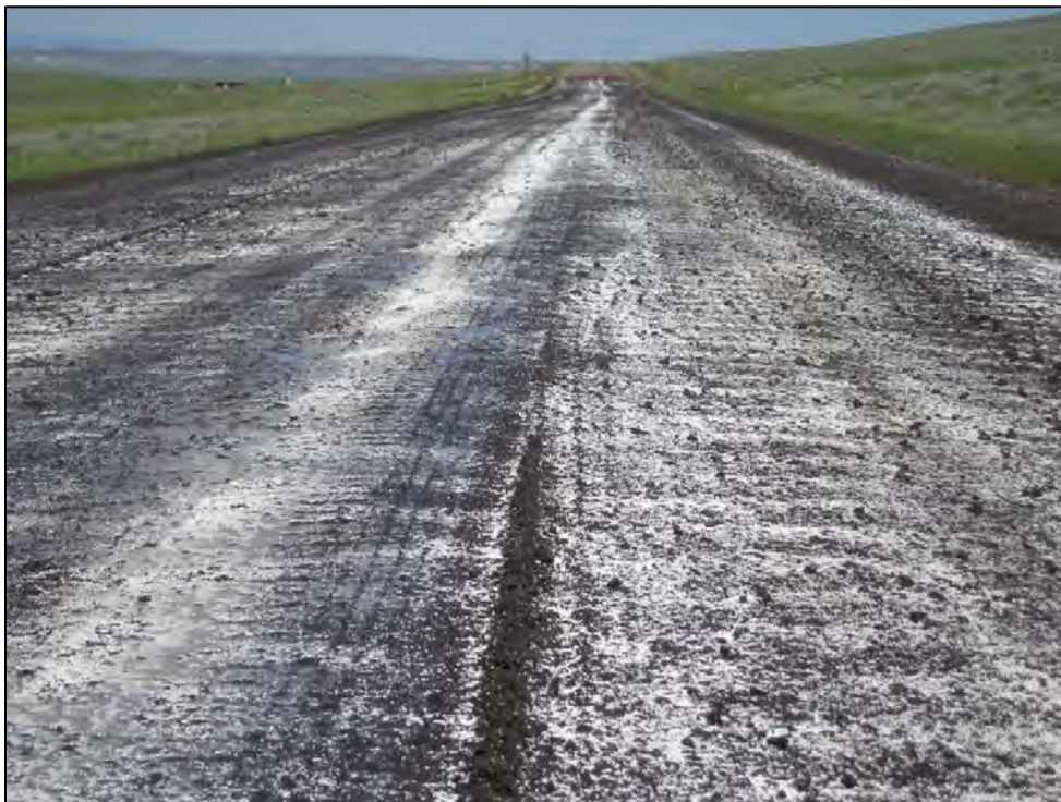
Figure 3.26 Calcium chloride flakes placed on damp RAP and aggregate blend on Johnson County's Schoonover Road, June 2008.
