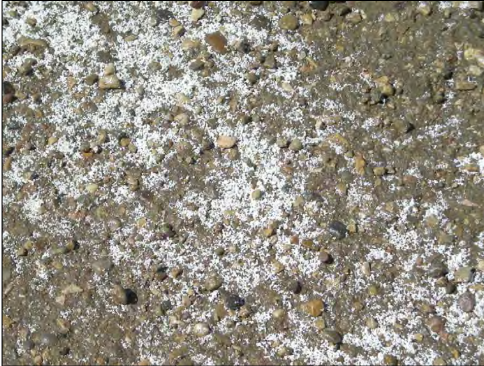
Figure 3.27 Close-up of calcium chloride flakes on Johnson County's Schoonover Road, June 2008.
