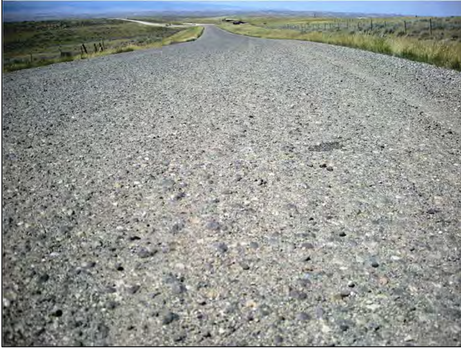
Figure 4.22 Road surface on Johnson County's Schoonover Road, segment S2 with RAP blend but no calcium chloride in August 2008, two months after RAP placement.
