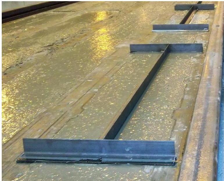
Figure 3.13 Steel bars cast in fresh concrete
