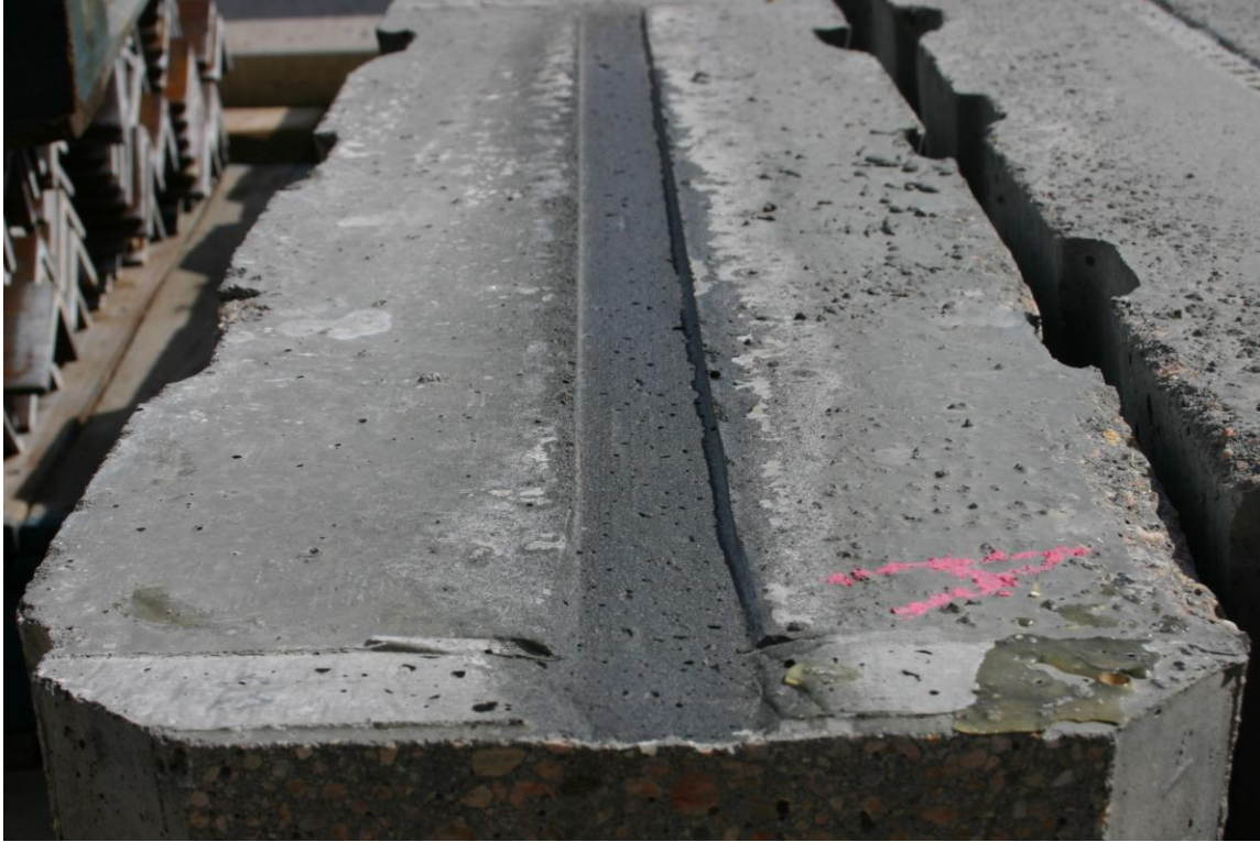
Figure 3.15 Notch created by steel bar inserts
