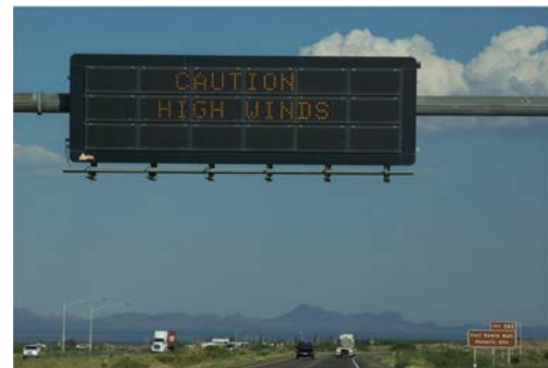
Figure AZ-2. Dynamic message sign with warning message.
