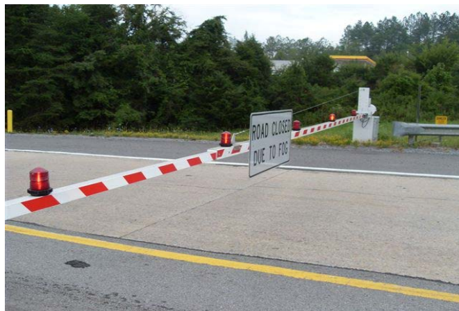
Figure TN-4. Swing gate.
