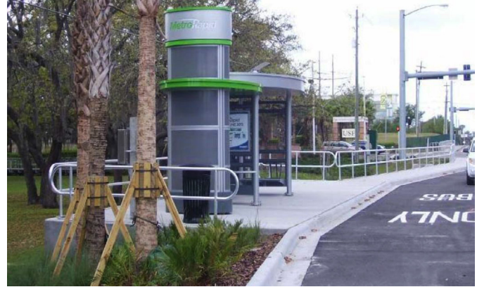
The MetroRapid bus rapid transit (BRT) is under construction in Tampa. Distinctive stops are an important feature in attracting riders to BRT.
