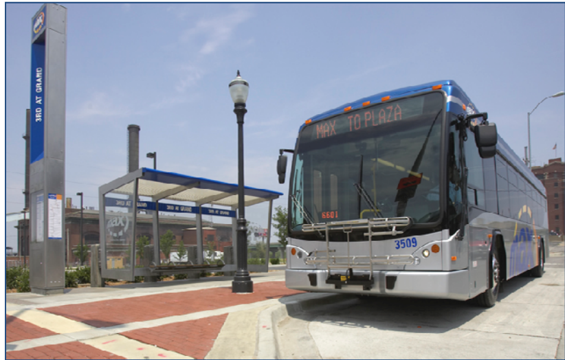
Figure 6 HealthLine Raised-Platform Median Station, Cleveland
