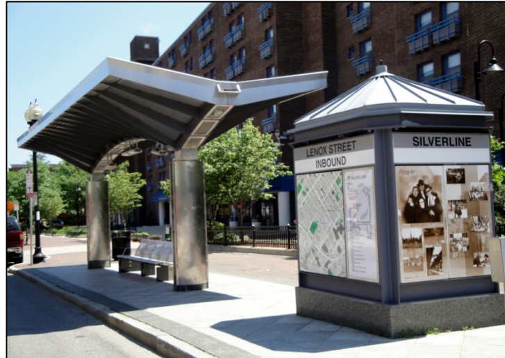
Figure 9 SilverLine Station and Travel Way, Boston
