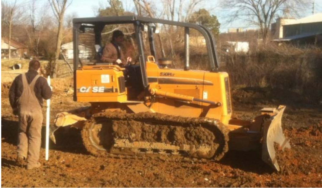
Figure 3.8. Case 560H tracked tractor use on the MBTC-3031 project.
