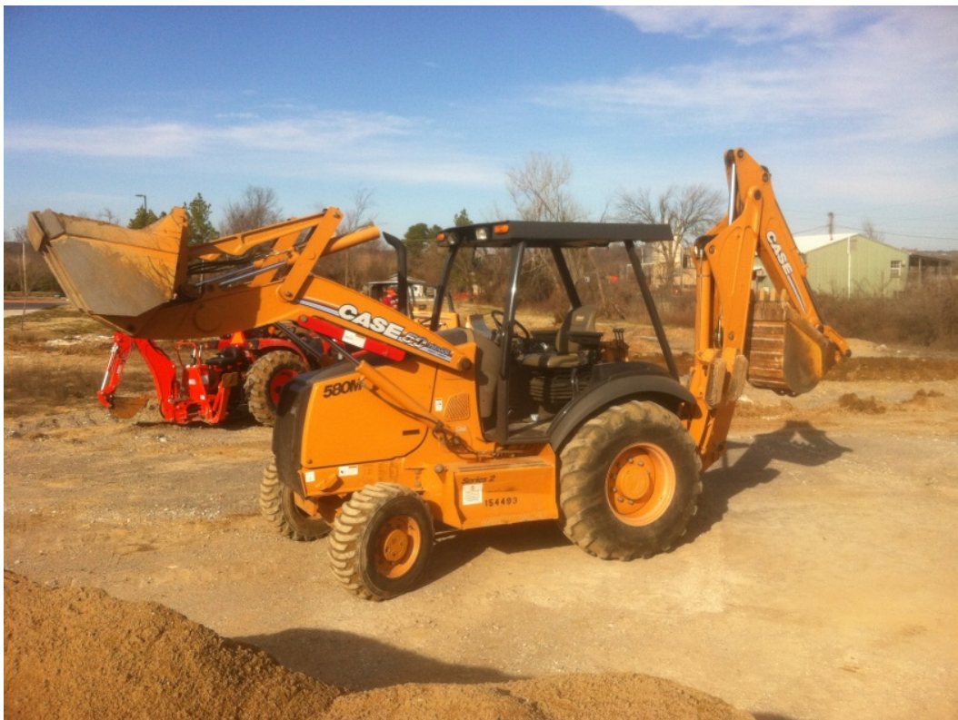
Figure 3.9. Case 580M backhoe loader used on MBTC-3031 project (Kioti utility tractor in background).
