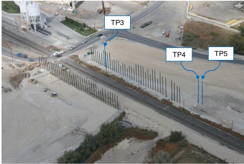
Figure 3.7: Piles for the Pioneer Crossing bridge over UPRR prior to wall construction.
