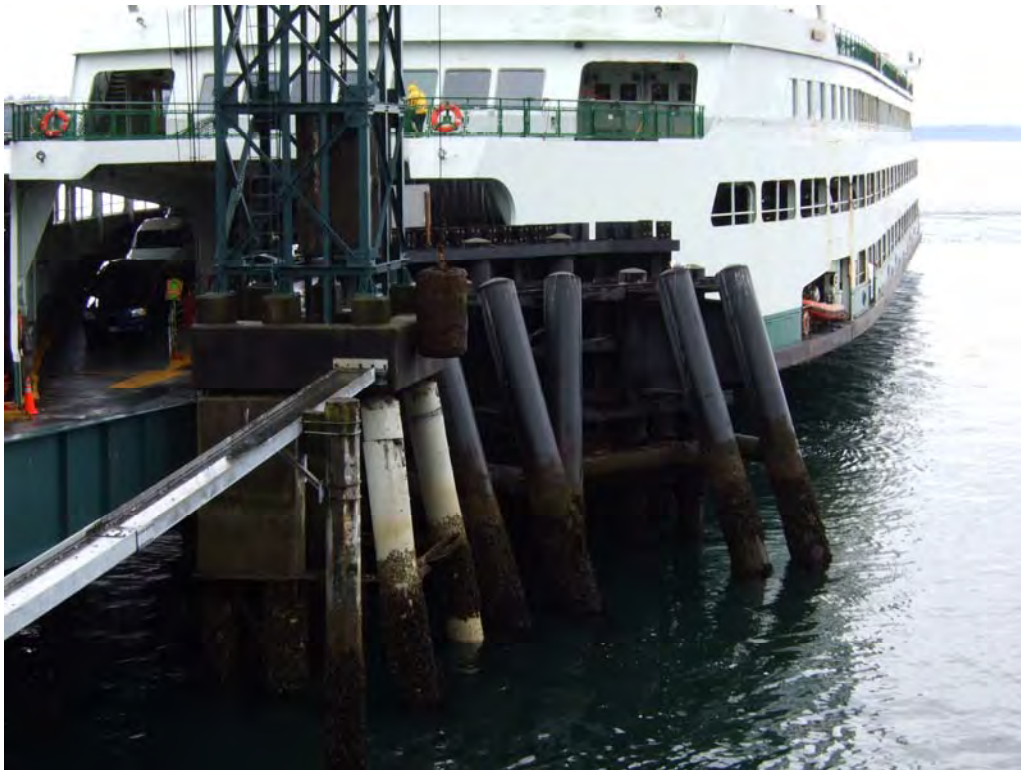
Figure 3: Seattle Ferry Terminal, Seattle, WA. (Wingwall supported by dark piling)
