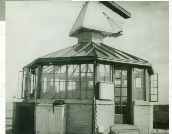
1930, first radio-equipped control tower, Cleveland Municipal Airport
