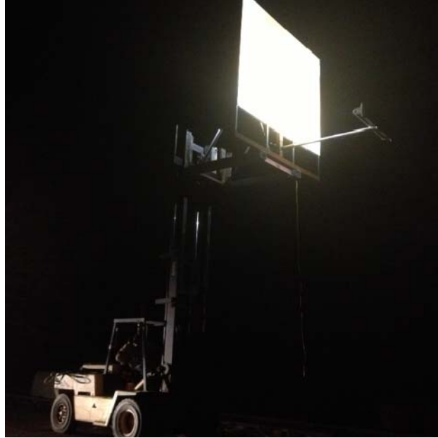
Figure 3.12 Sign Structure Lifted by a Forklift
