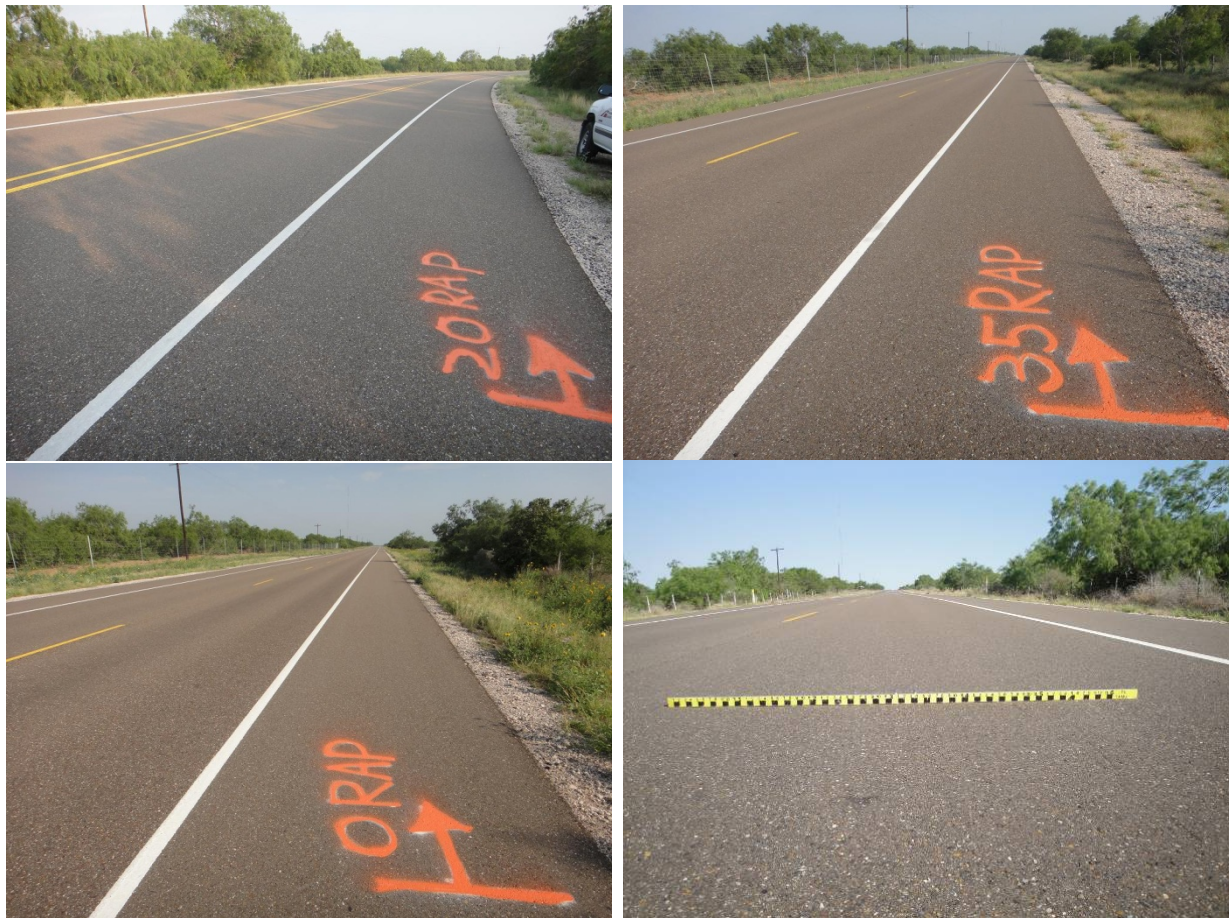
Figure 4. RAP Test Sections on FM1017 on May 25, 2012.
