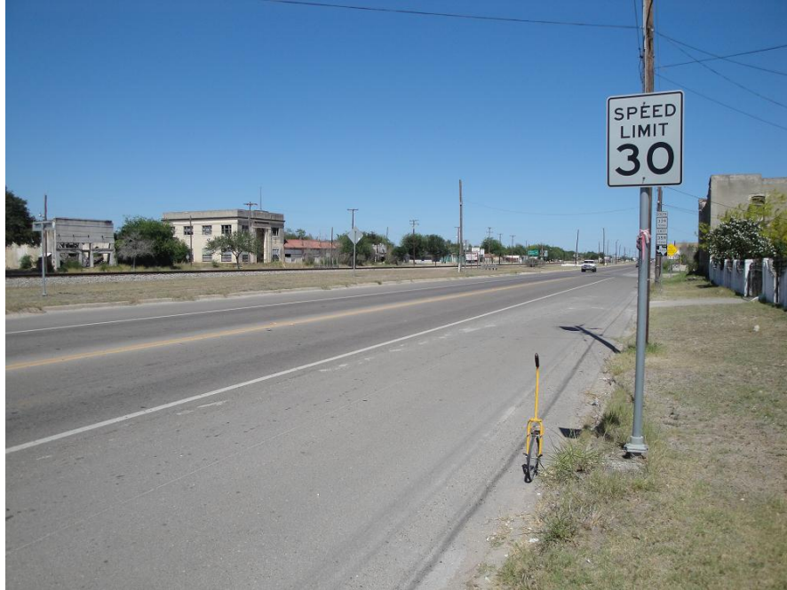
Figure 6. Perfect Condition of RAP/RAS Test Section on SH359.
