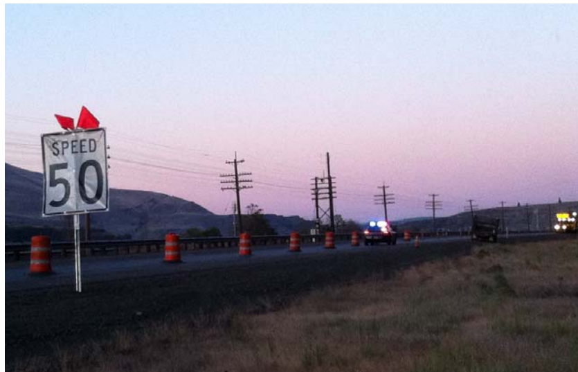
Figure 3.11: OSP Parked at the End of Taper with Lights On
