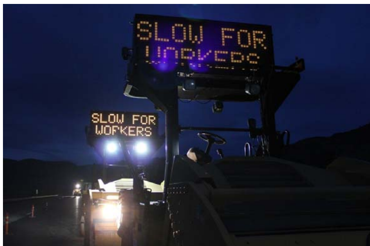
Figure 3.10: PCMS on Rollers for I-84 Case Study Project
