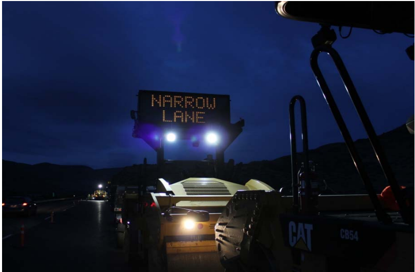
Figure 2.10: PCMS on Roller
