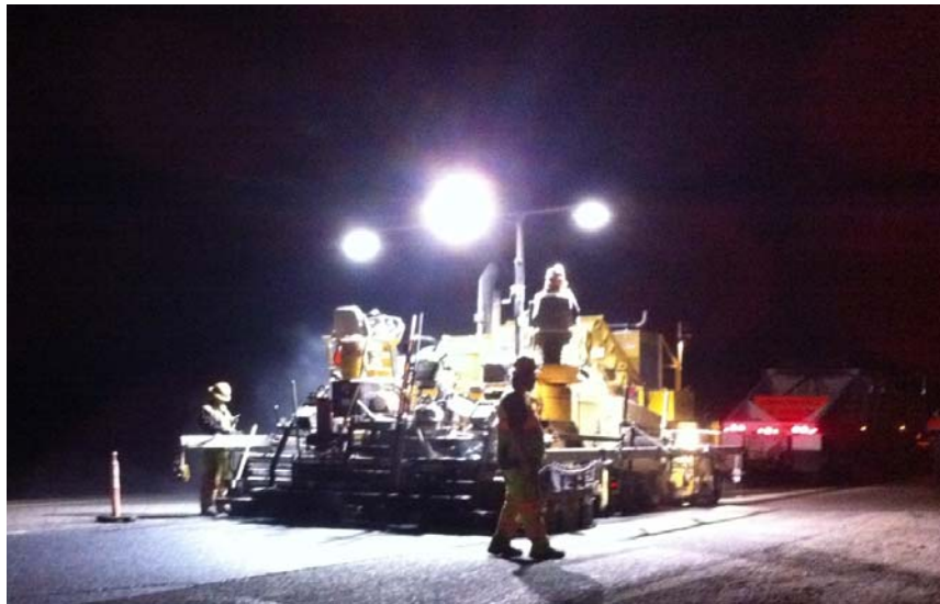
Figure 4.1: Paver for I-84 Project
