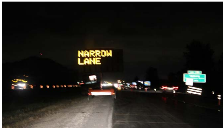
Figure 3.17: PCMS Sign on Trailer for I-5 Case Study Project
