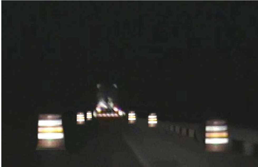
Figure 3.14: Drums on Both Sides of Travel Lane
