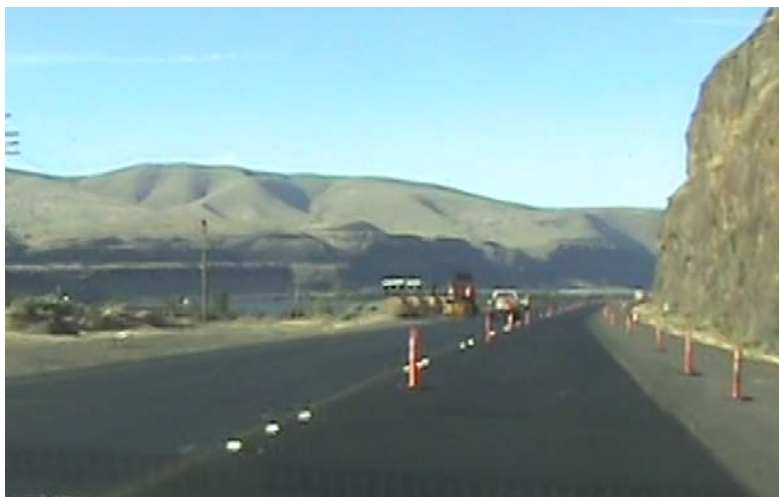
Figure 3.13: Tubular Markers on Both Sides of Travel Lane
