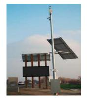
Figure 1. Typical sensor array for CA's fog detection and warning system
