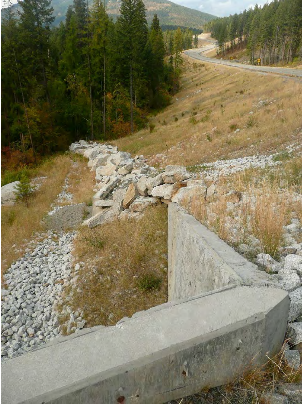
Exhibit 7. Wing wall at wildlife underpass and connection to large boulders, substituted for wildlife exclusion fence on west-side of US 95, near Bonners Ferry, Idaho. (copyright: Tony Clevenger)
