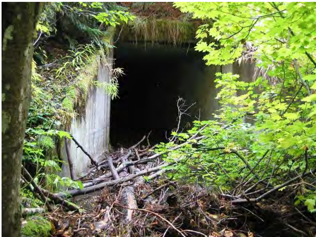
Price Creek Culvert north entrance. (Photo: WTI)
