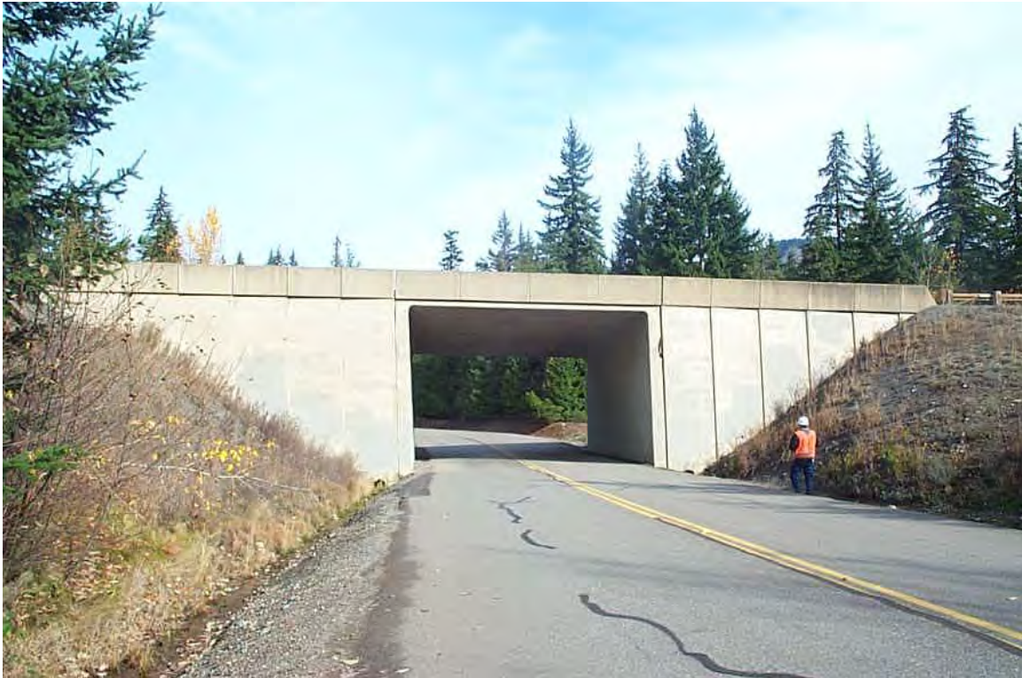
Sparks Road Bridge South. (Photo: WSDOT)
