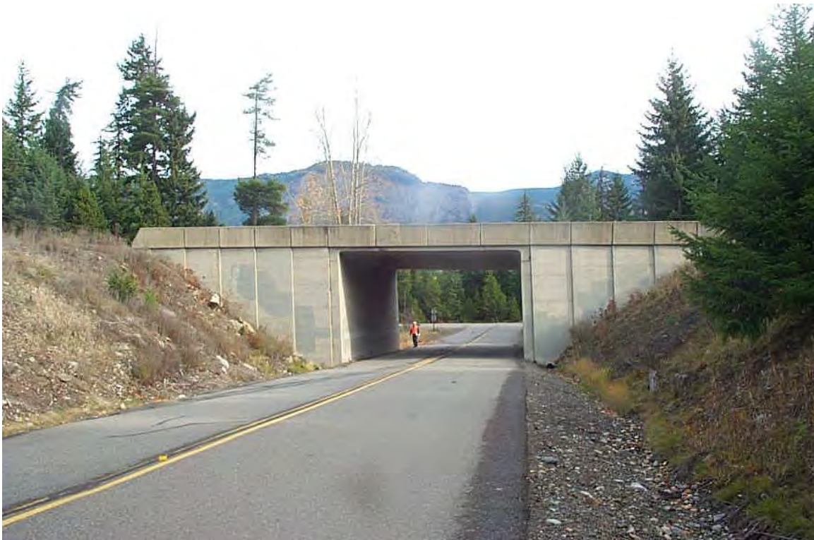
Sparks Road Bridge North. (Photo: WSDOT)
