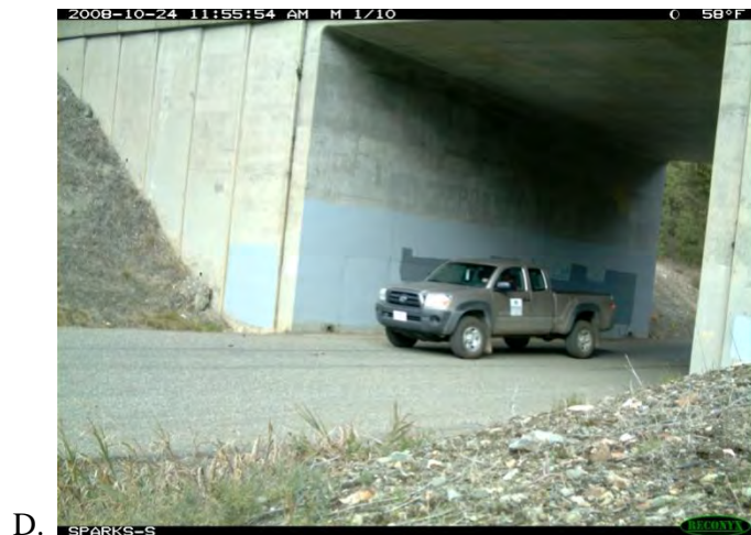
Figure 3.4. “Faux” electrical housing containing remote camera deployed at the Sparks Road Bridge South. Various images show housing (A), aim of camera (B), view from under the bridge with arrow pointing to camera box (C), and sample photo of WTI field vehicle (D). (Photos: R. Long /WTI)
