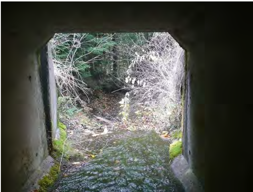
Cedar Creek Culvert north entrance. (Photo: WTI)
