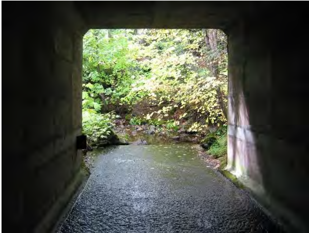
Price Creek Culvert south entrance. (Photo: WTI)
