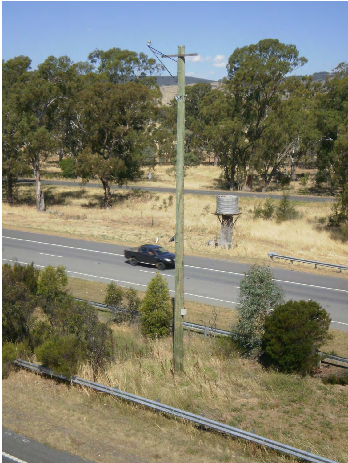
Figure. 5.10. Glider pole deployed in the median of a split highway in New South Wales, Australia (Photo: Rodney van der Ree)
