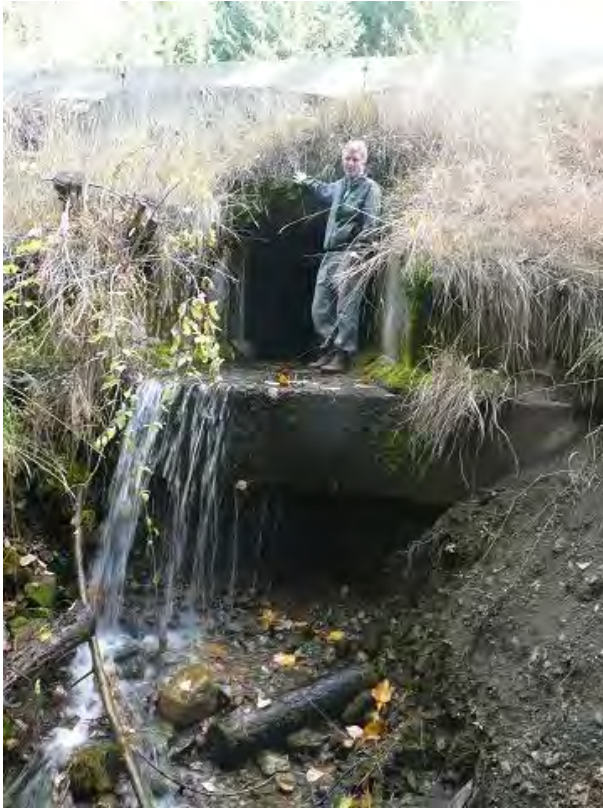
Cedar Creek Culvert south entrance with dropoff. (Photo: WTI)
