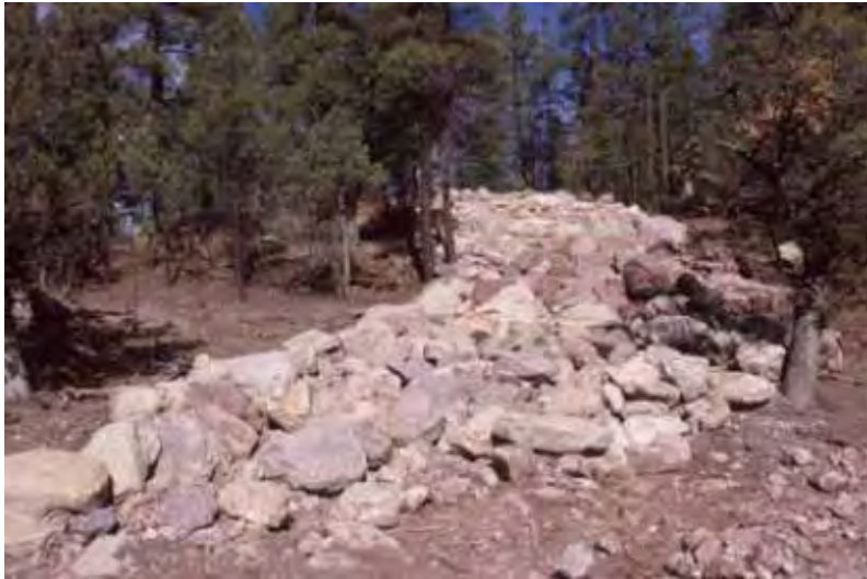
Exhibit 9. Large boulders placed in the right of way as a barrier to elk and deer along State Route 260 in Arizona (copyright: Marcel Huijser).
