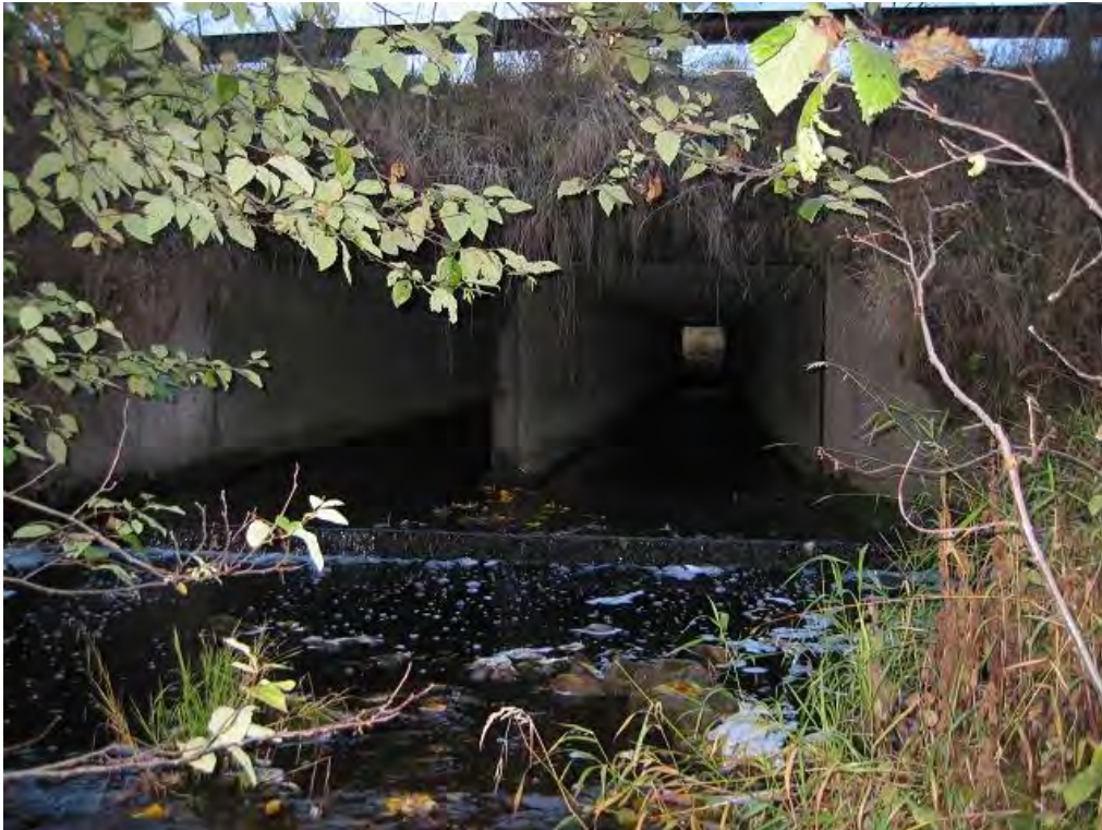
South entrance of paired Swamp Creek Culverts. (Photo: WTI)
