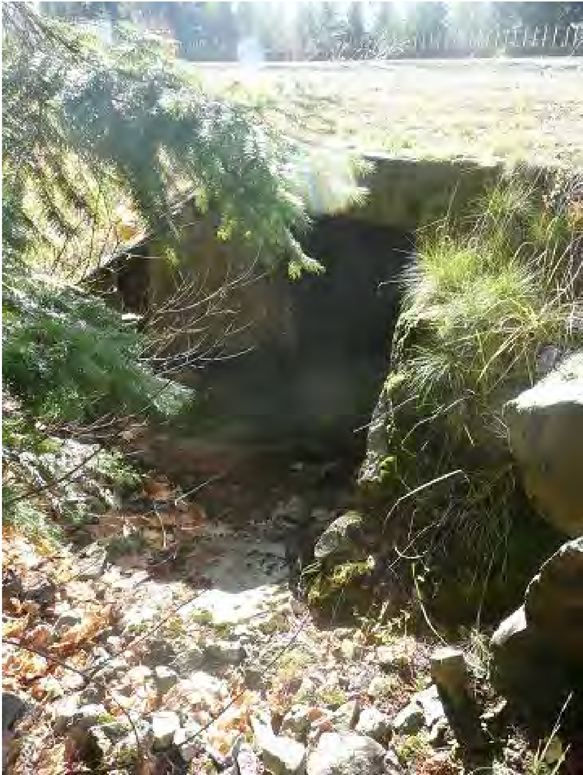
Unnamed Creek Culvert north entrance. (Photo: WTI)
