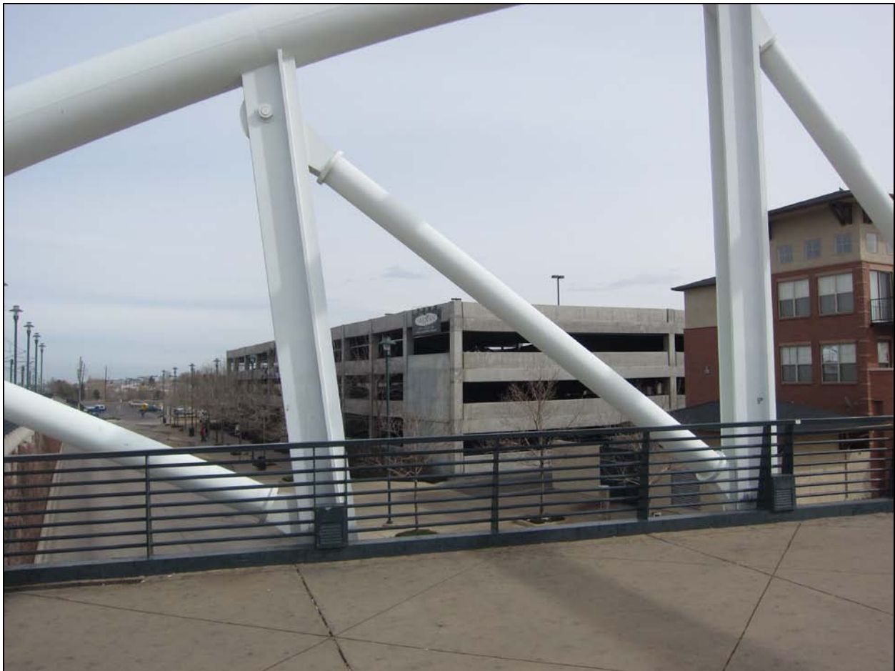
Figure 2.14: Example of concrete multi-storey parking lots near LRT station, Denver, Colorado
