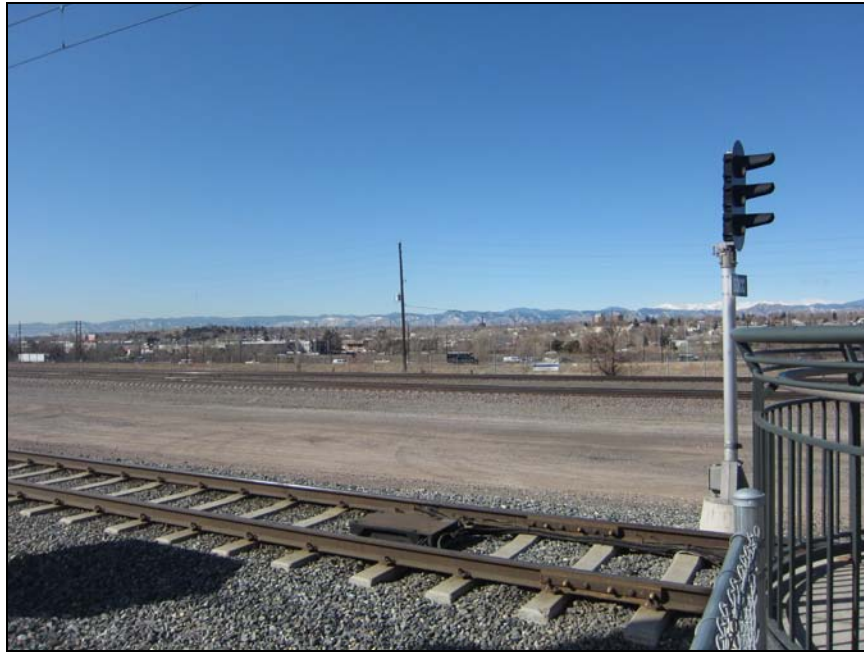
Figure 2.6: LRT alignment next to a heavy rail track.
