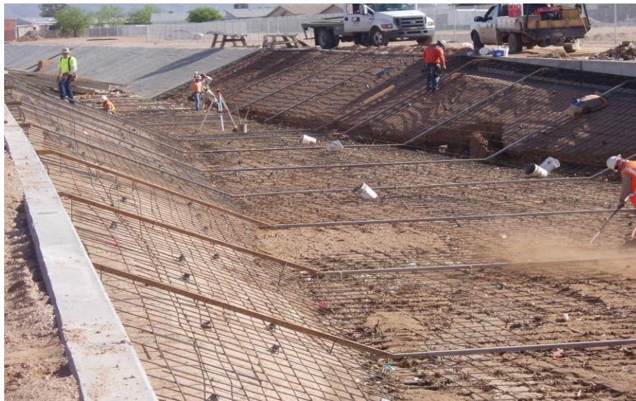
Figure 5. Cleanup Operation for a Canal during Construction When an Occasional Rainfall Results in Debris Accumulation and Grade Changes of the Prepared Base. Photo Courtesy of Rich Shelly, Pulice Construction Co.
