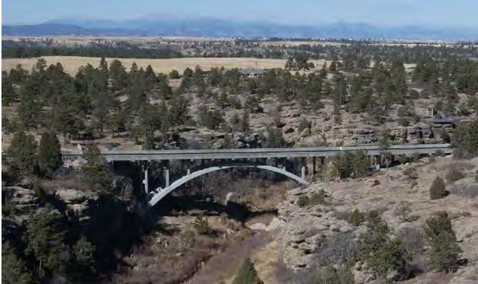
Figure 2.2 Castlewood Canyon Bridge (Mohseni, CDOT)
