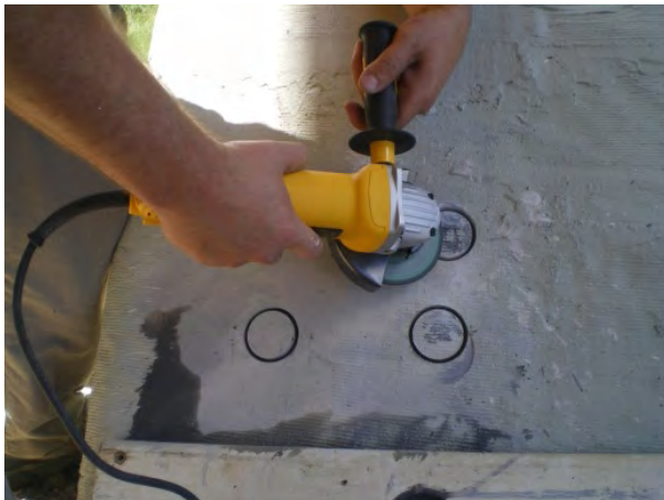
Figure 3.8 Removing the acrylic paint later before adhering the aluminum pucks
