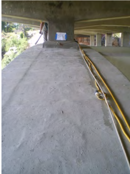
Figure A14. Bay 5NE
