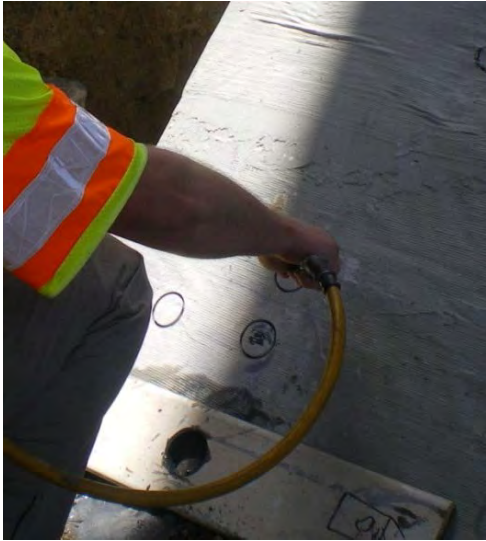
Figure 3.7 Removing water and debris from core cuts
