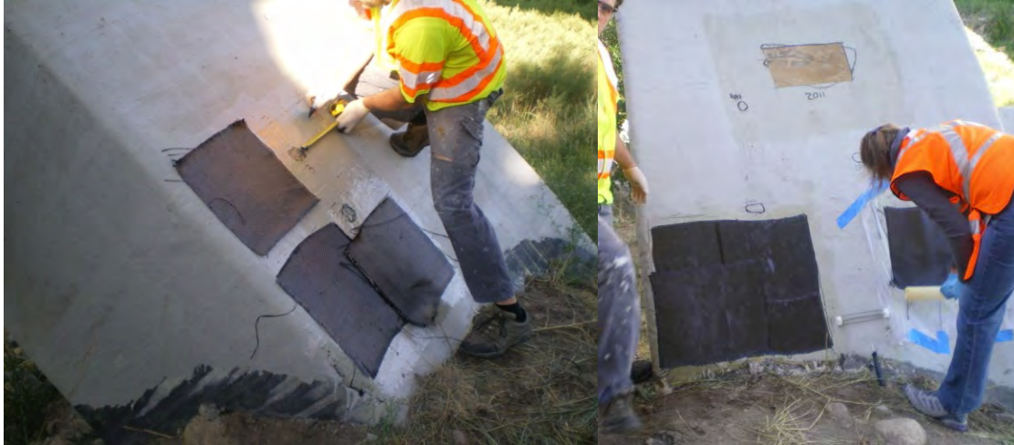
Figure 3.26 Allocating fabric for repair and applying the second layer of CFRP to the area of pull-off tests on the east arch
