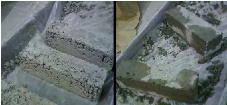
Figure 6.9 Concrete beams before (left) and shortly after (right) patching
