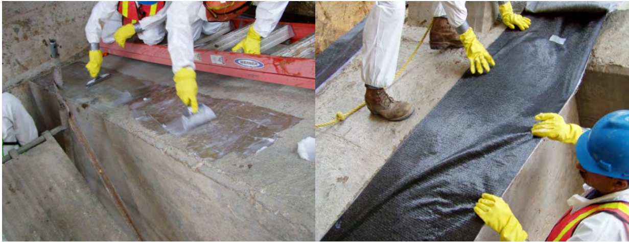
Figure 2.10 Fyfe’s Tyfo® S Epoxy resin (likely with glass fibers as a filler) being applied to the extrados of an arch and installation of saturated unidirectional CFRP fabric, Tyfo® SCH-41 (Mohseni, CDOT)
