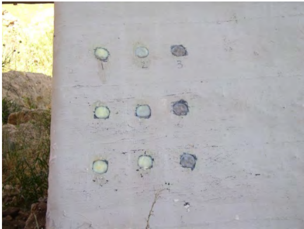
Figure 3.24 Epoxy filled holes following the pull-off tests
