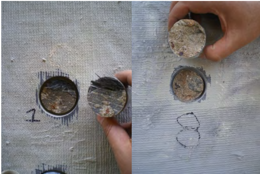
Figure 3.15 Failure Modes B and F: cohesive failure in FRP laminate, and mixed cohesive failure in substrate and adhesive failure at the adhesive/substrate interface, respectively (on left), Failure Mode G: cohesive failure in concrete substrate (on right)
