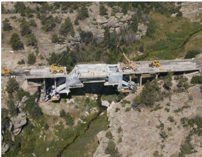
Figure 2.6 Systematically replacing the bridge deck (Mohseni, CDOT)
