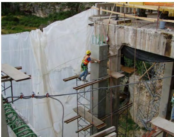
Figure 2.7 Placing the new spandrel columns adjacent to the existing columns (Mohseni, CDOT)
