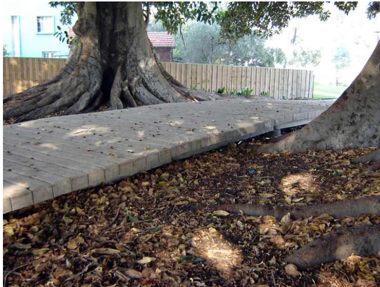
Figure 3-7: Precast Concrete Boardwalk (Source: PermaTrak, 2012)
