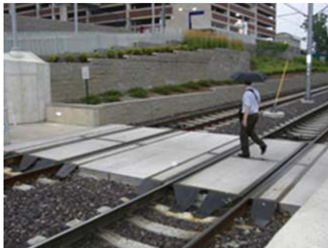
Figure 3-6: Precast Concrete Pedestrian Panels at Light Rail Station (Source: Century Group, 2012)
