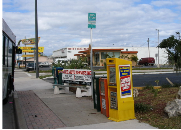
(b) Depth of the B&A area barely meets the minimum 8' requirement; however, it is obscured by a bench and paper kiosks.
