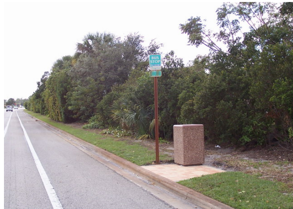
(d) Although there is not a sidewalk, the shoulder may serve as the accessible path; however, the B&A pad does not meet the size requirement and is also obscured by a trash can.
