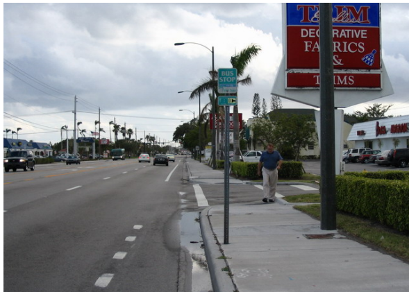
(c) Sidewalk does not meet the minimum depth requirement of 8' and it is also obscured by a pole.
