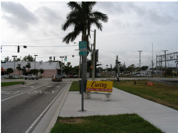
(c) B&A pad suitable for both front- and rear-door boarding and alighting (but with partial obstructions).
