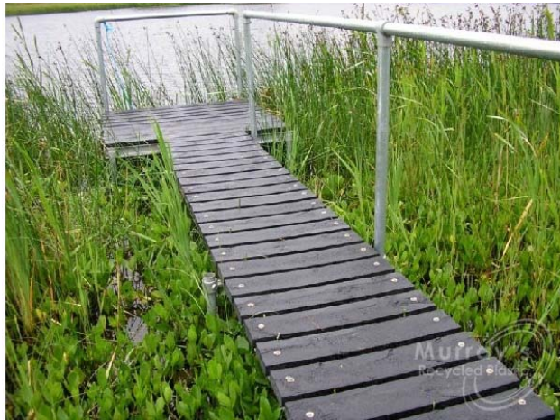
Figure 3-18: Plastic Lumber (Source: Murray's Recycled Plastic, 2012)
