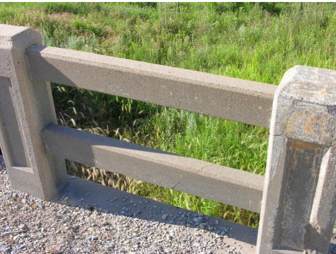
Figure 26. Examples of Concrete Post and Rail System
