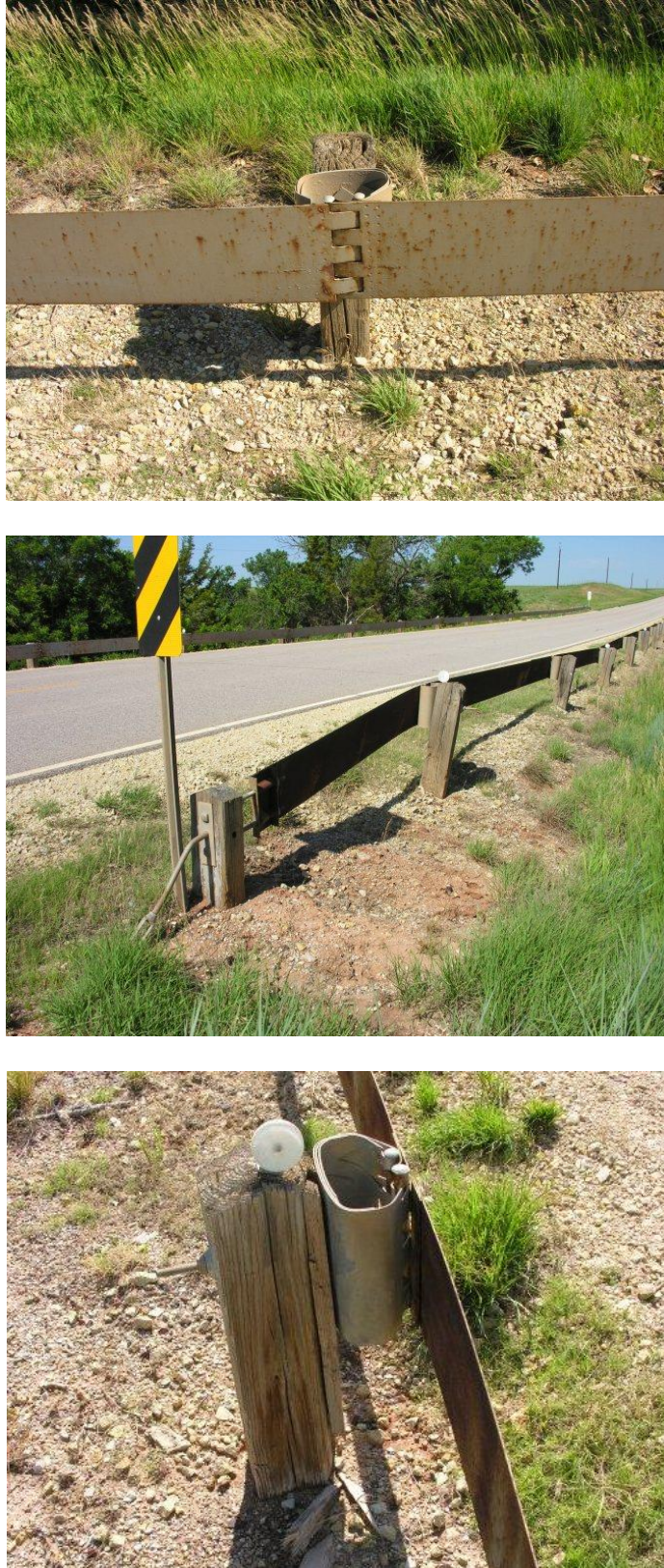
Figure 24. Examples of Flat-Panel Systems
