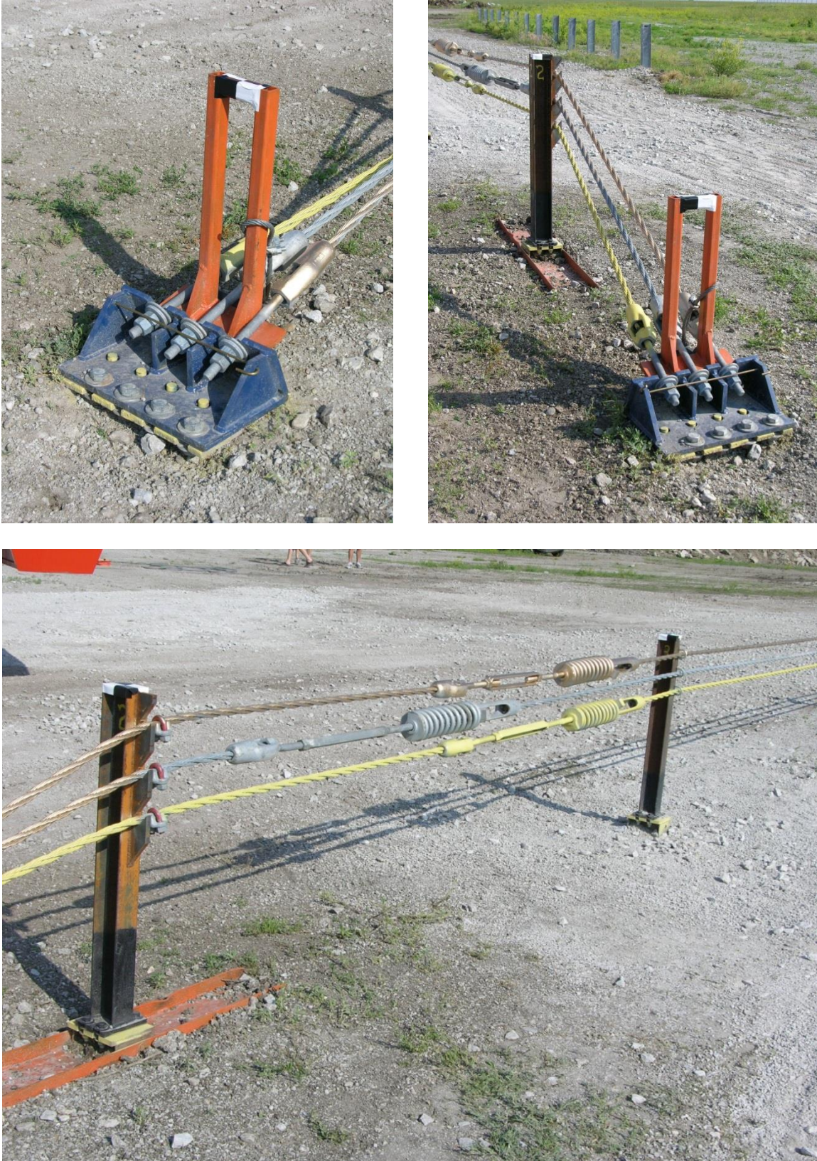
Figure 4. Generic Low-Tension Cable End Terminal
