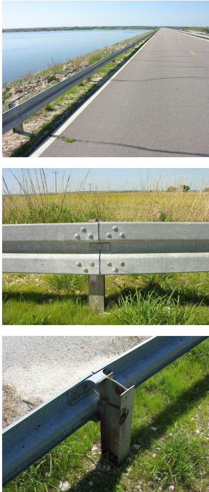
Figure 25. Examples of Channel Rail Systems
