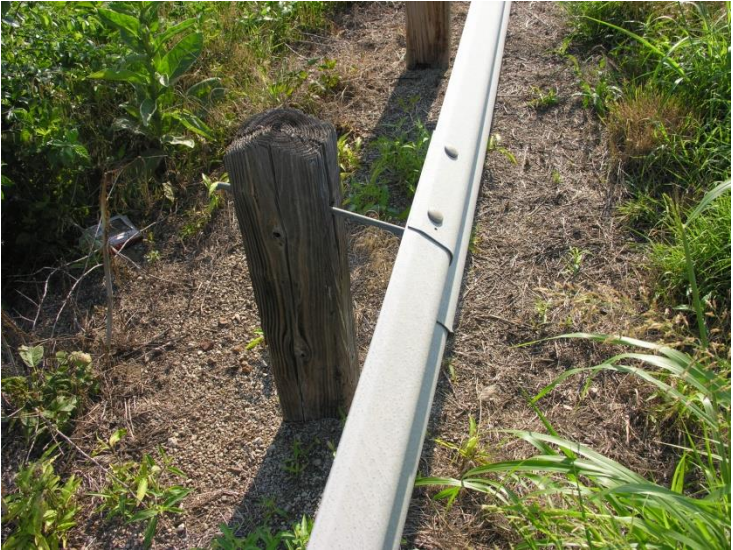
Figure 20. Examples Missing Blockouts in Existing Systems
