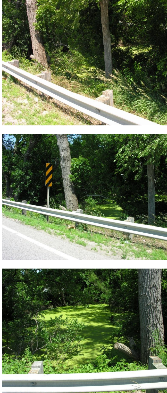
Figure 7. Examples of Shielded Roadside Trees and Pond
