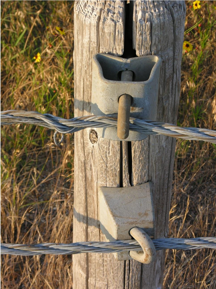
Figure 22. Examples of Cable Barrier Systems
