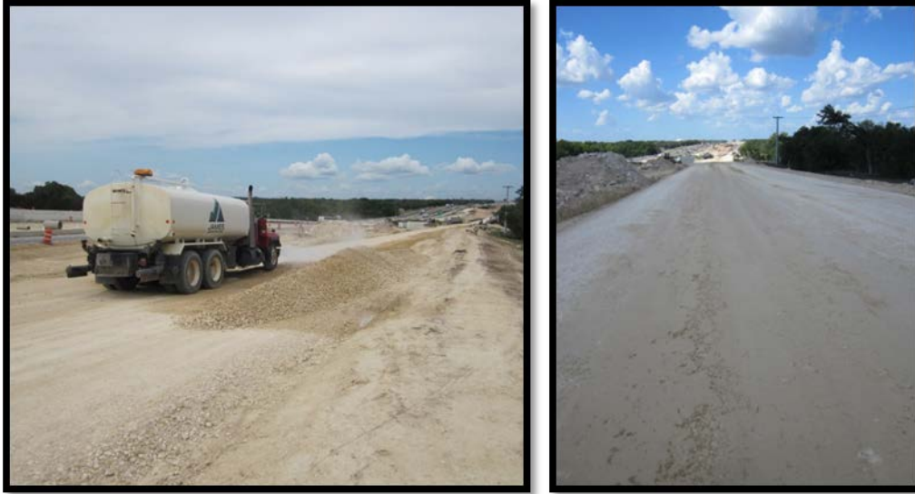
Figure 3.18. Processing and Finished Base on Field Test Site.
