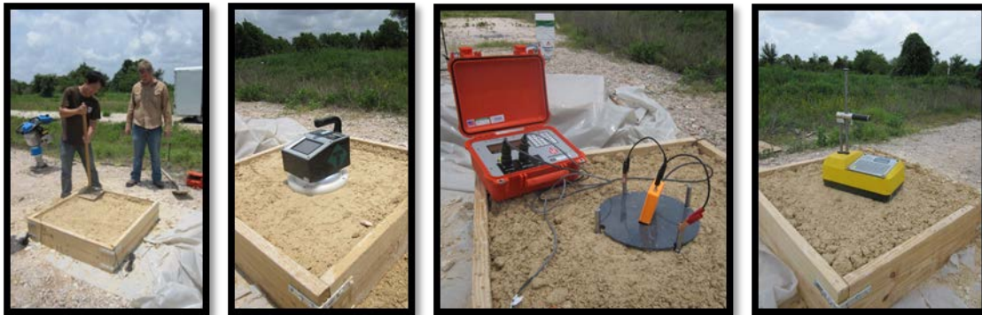
Figure 3.3. Smoothing and Testing with SDG, EDG, and Nuclear Gauge on Test Box.
