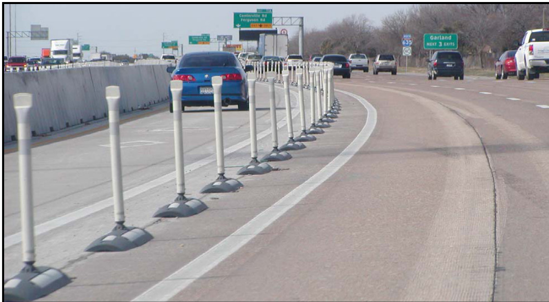
Figure 17. Curb-Pylon Implementation on IH 635 in Dallas (8).
