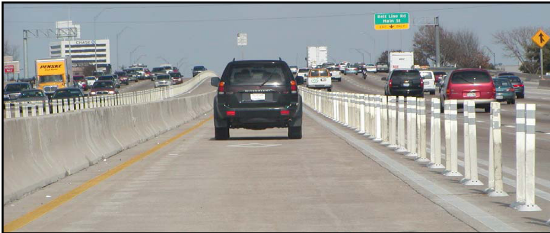
Figure 15. Curb-Pylon Implementation on US 75 HOV in Dallas (6).
