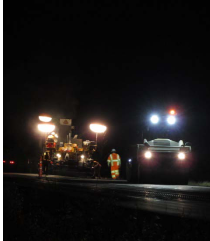
Figure 6. Paver and Roller in Bryan-College Station.
