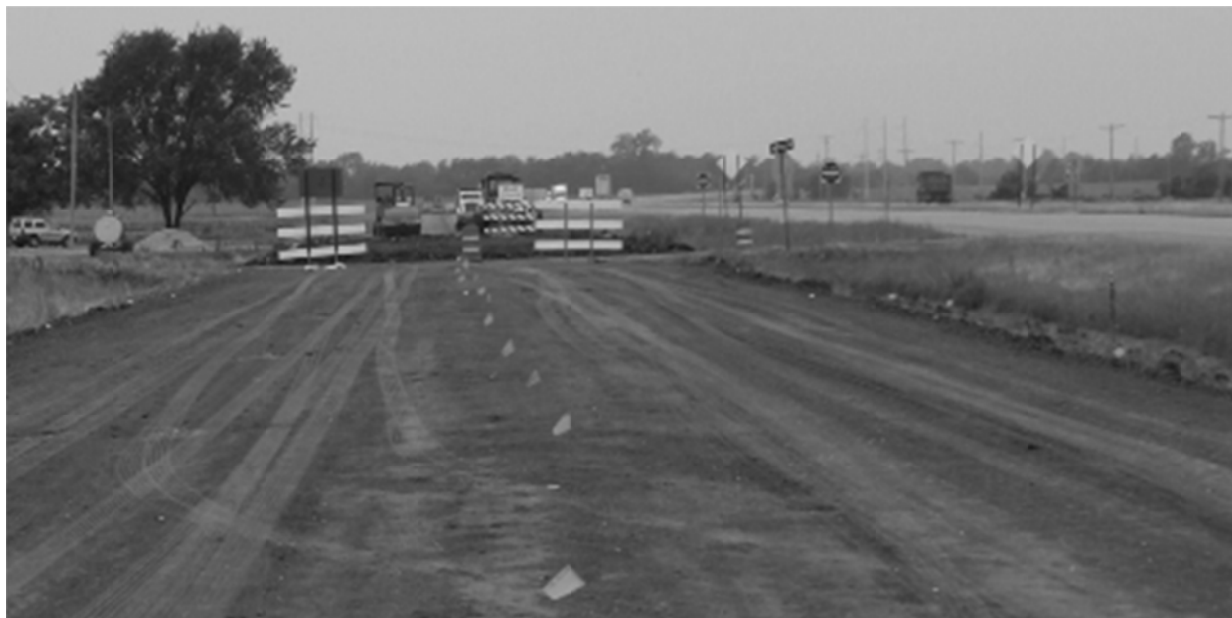
Figure 3.10. Finished cut subgrade (Howard 2006).
