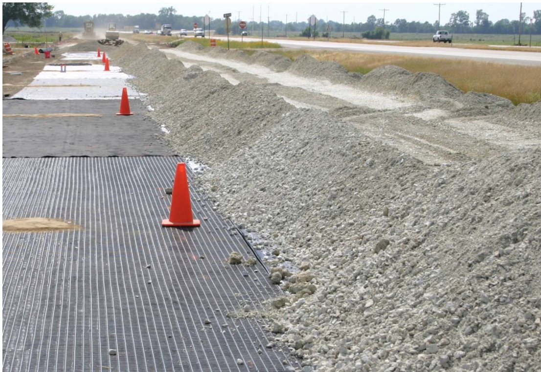
Figure 3.17. Base course placement on non-instrumented lane (Howard 2006).
