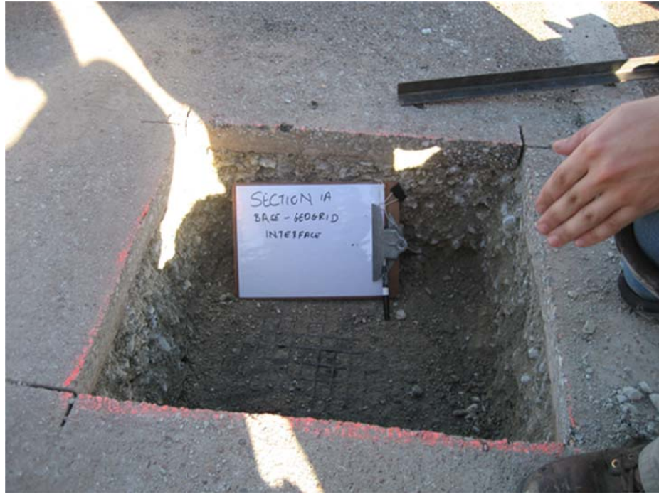
Figure 6.9. Subgrade-geosynthetic interface of Section 1A (Mirafi geogrid).
