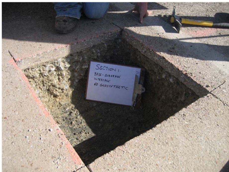
Figure 6.8. Base-subgrade interface of Section 1 (no geosynthetics).
