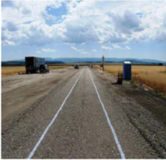
Figure 2.6. Full-scale field testing (Cuelho and Perkins 2009).
