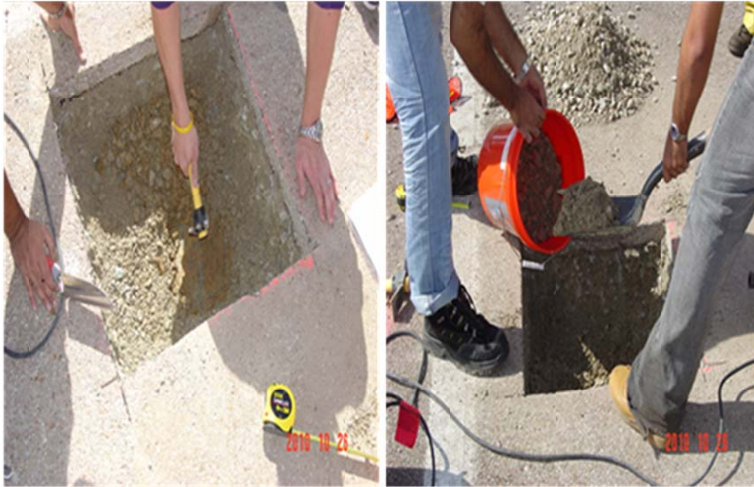
Figure 6.7. Base layer excavation and sampling at Section 2.
