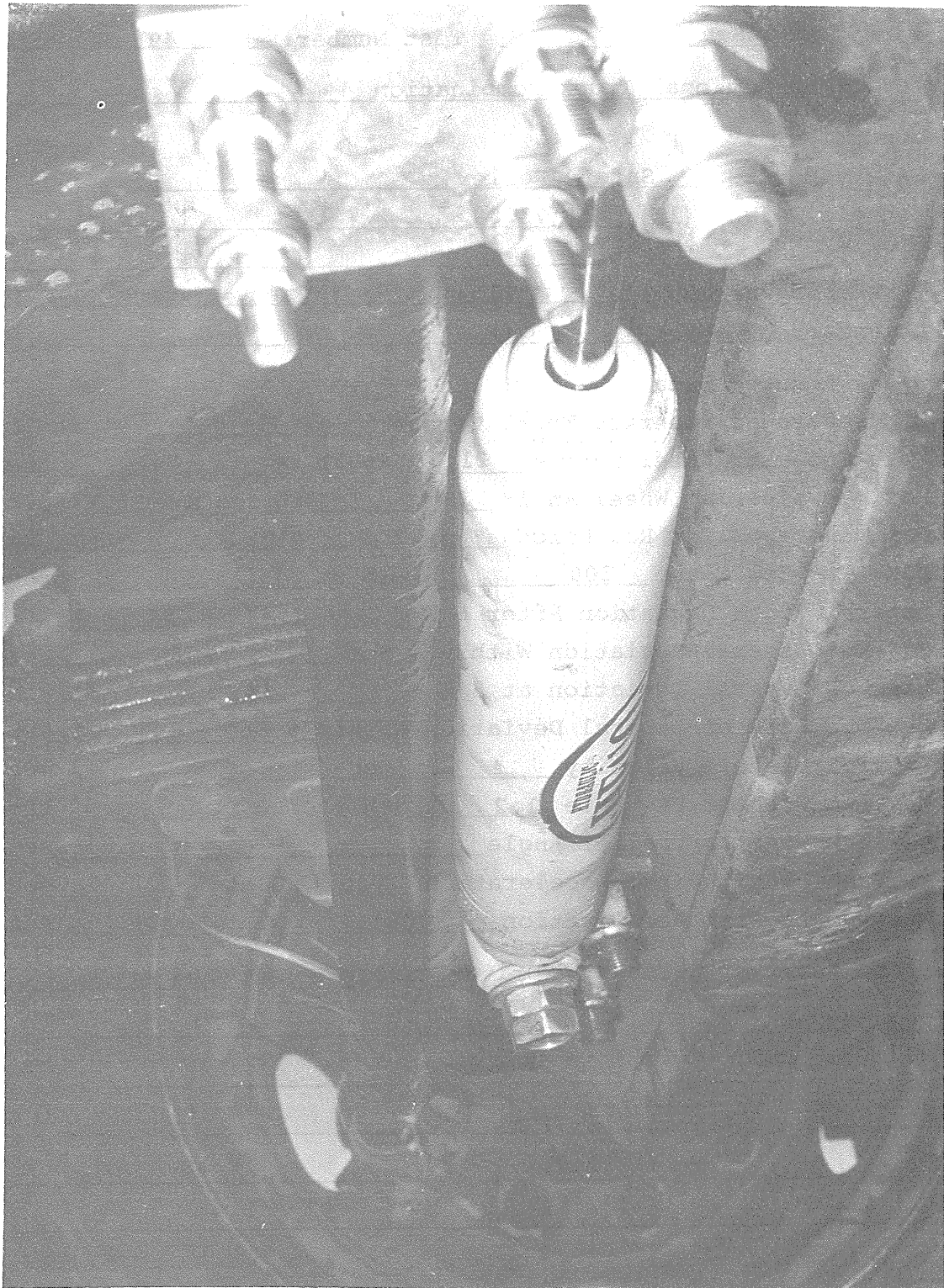
Figure 6-44. Pre-test View of HECO Device as Seen From Center of Tie Rod.
