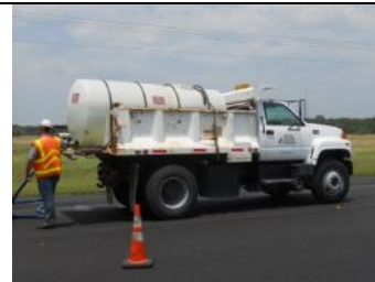
Water truck for filling the rollers water reservoir
