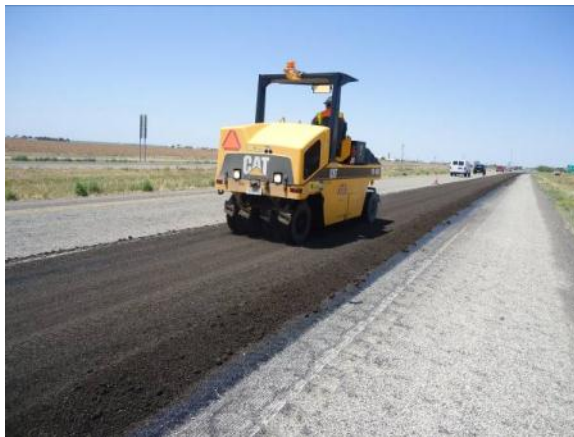
Step 4: Finishing up the surface with a pneumatic compactor.
