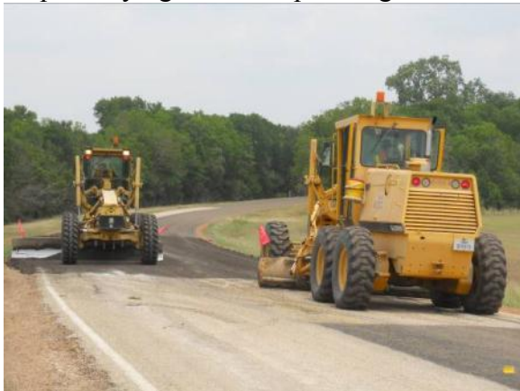
Step 6: Distributing the patching mix along the surface using two facing blades. Each blade patches over a single lane with overlapping to ensure smooth feathering over the center line. With dual blades this operation can be completed in shorter period of time allowing faster opening to traffic.
