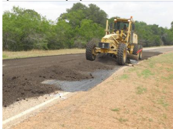
Step 6: Distributing the patching mix along the surface using two facing blades. Each blade patches over a single lane with overlapping to ensure smooth feathering over the center line. With dual blades this operation can be completed in shorter period of time allowing faster opening to traffic.
