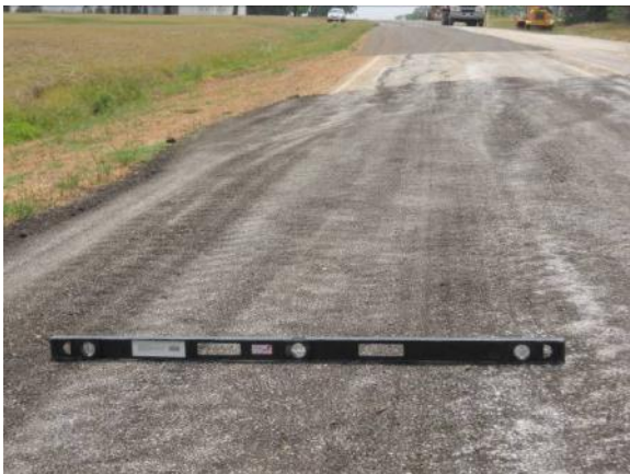
Step 8: Evaluating the cross slope by visual inspection using a straight edge at various spots. Driving on the finished surface also provides a feedback on the longitudinal slope and the ride smoothness.
