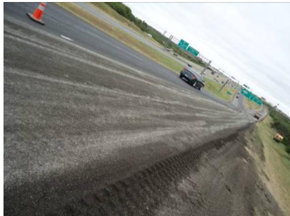
Step 8: Finishing up the surface with steel wheel compactor to compact the multiple layers and provide a smooth surface. Blade the excess from the side to for a smooth slope along the shoulder.
