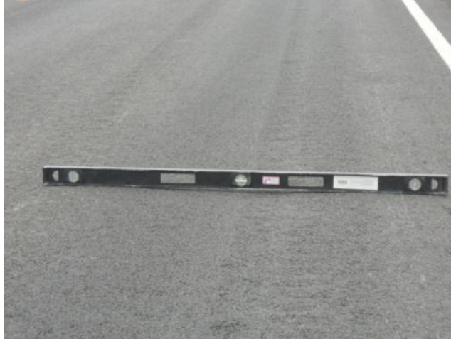
Figure 4-8. Rutting Reappeared in FM 979 after One Year of Level-up Patching due to Soil Movements.
