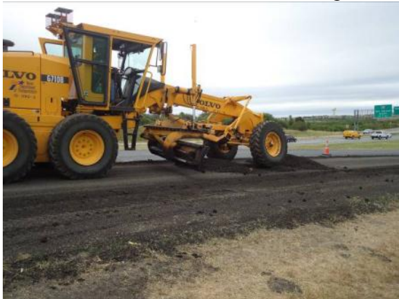
Step 5: Blading the mix in 0.5 inch thickness with multiple back-and-forth passes.
