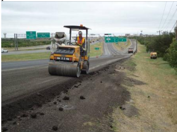
Step 8: Finishing up the surface with steel wheel compactor to compact the multiple layers and provide a smooth surface. Blade the excess from the side to for a smooth slope along the shoulder.
