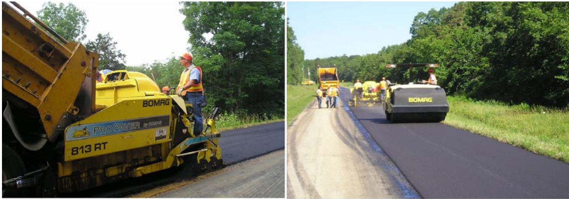
Figure 2-1. Level-up Patching Using Laydown Paver and Roller Compactor (MoDOT 2006).
