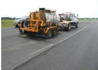
Asphalt Distributor for tack coat application
