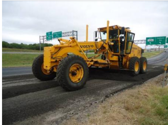
Step 5: Blading the mix in 0.5 inch thickness with multiple back-and-forth passes.
