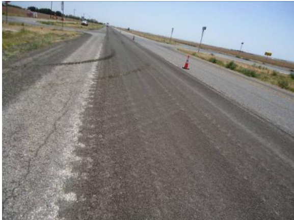
Step 5: Inspecting the level-up patching by the supervisor.
