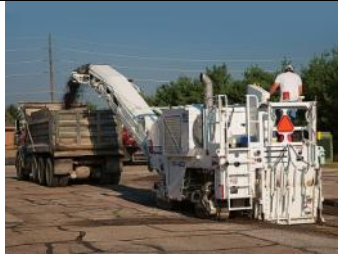
Roto-Mill machine for full-lane milling
