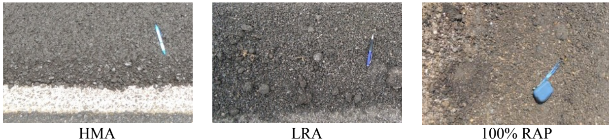
Figure 4-7. Examples of the Surface Mixes Used in Level-up Patching.
