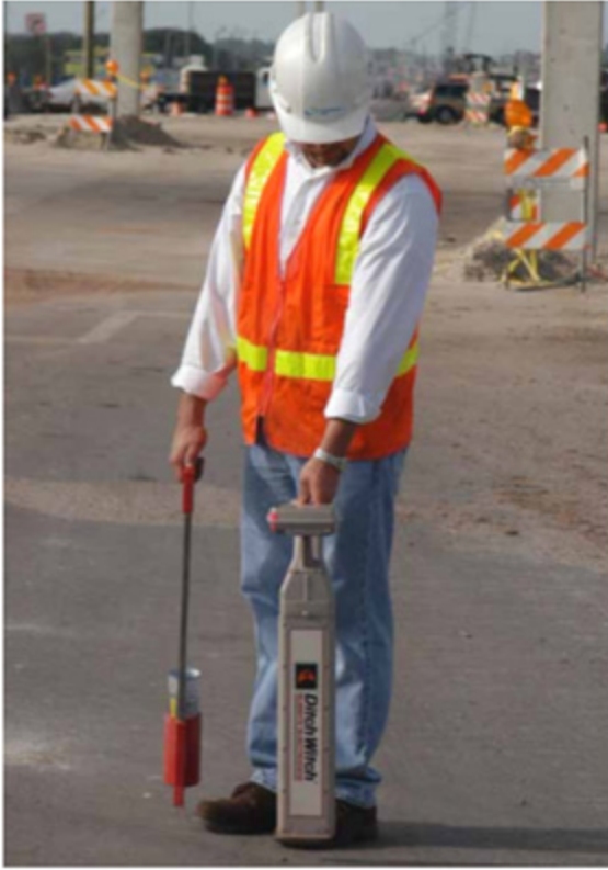
QLB data collection using pipe locator.
