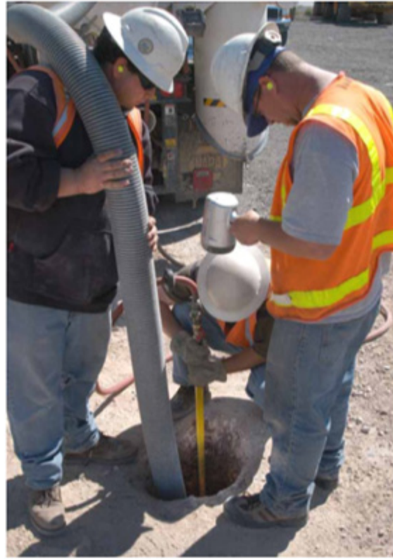
QLA data collection using vacuum excavation.
