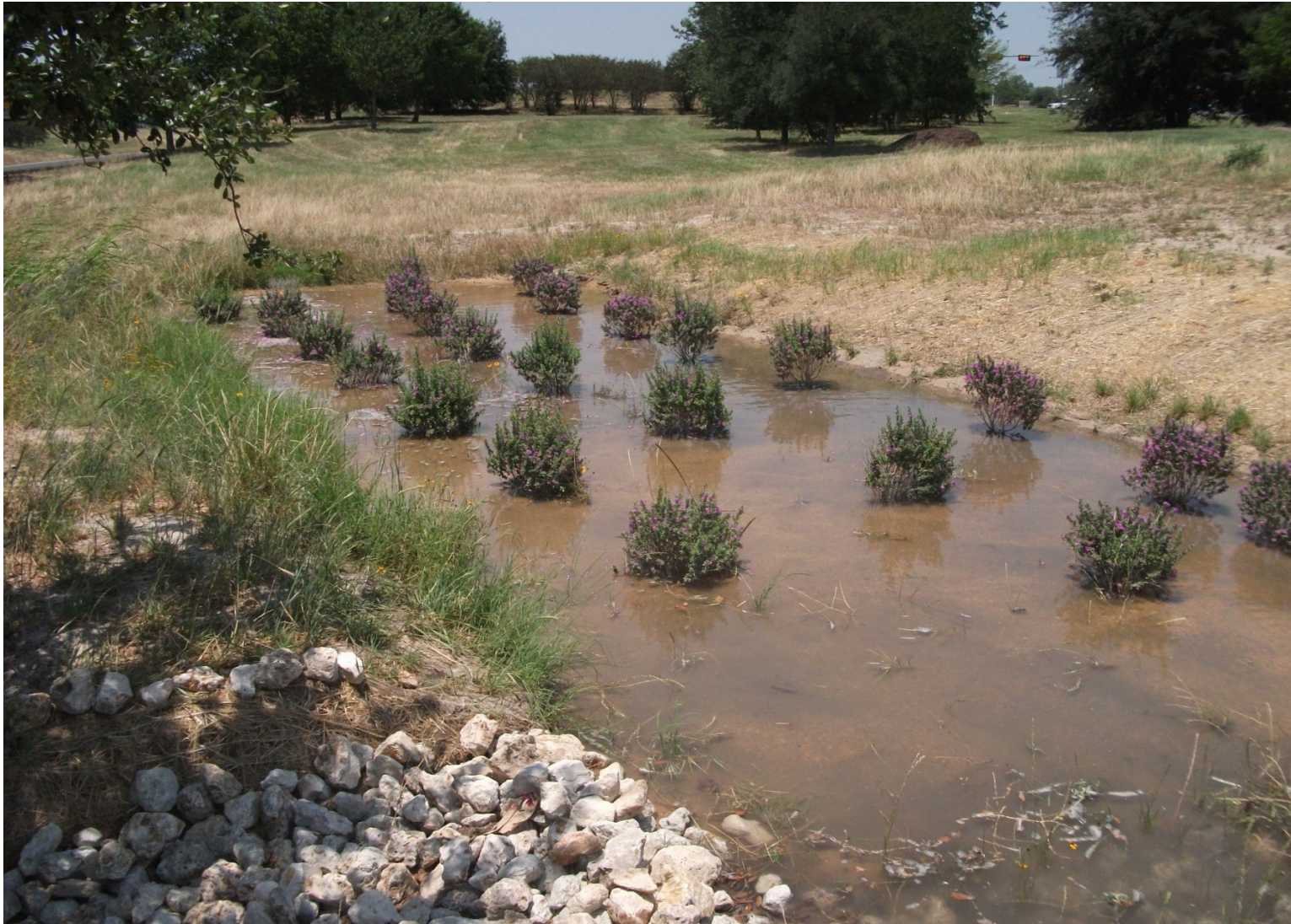
Figure 8. Flood Irrigation of Bioretention Cell (Photo Taken in June 2011).
