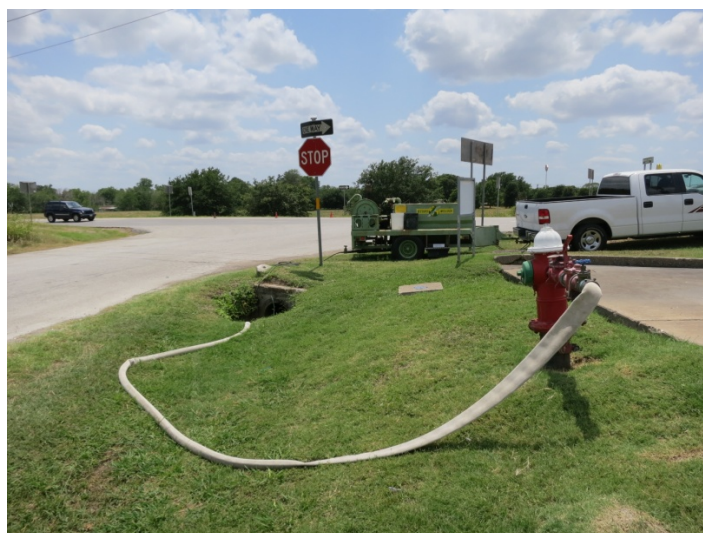
Figure 15. Fire Hydrant and Hydro-Seeder near Grass Swale Inlet.
