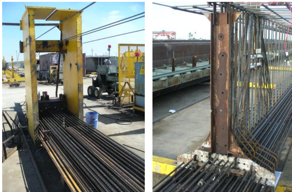
Figure 12–Jacking frame (left), and steel bulkhead (right).
