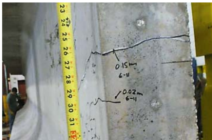
Figure 63–Web crack measurements (view from end of specimen)
