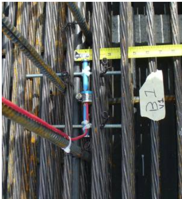
Figure 37–V gage installation (view from above)
