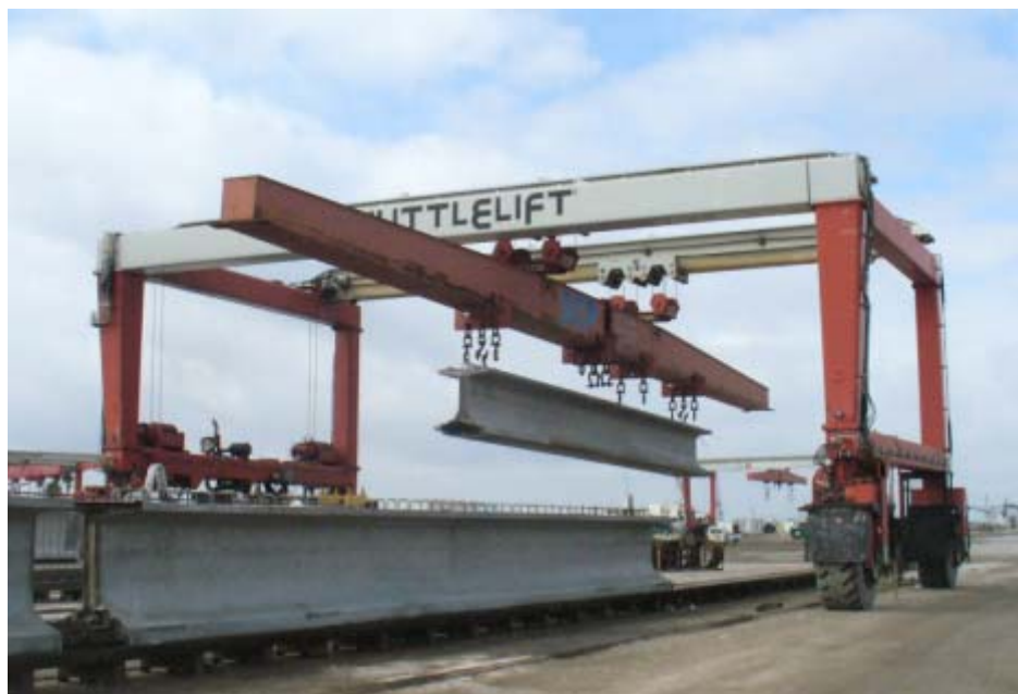
Figure 29–Test girder lifted by crane
