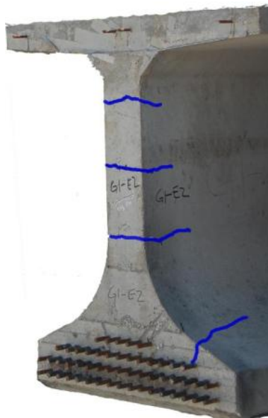
Figure 69–Web splitting and flange splitting cracks
