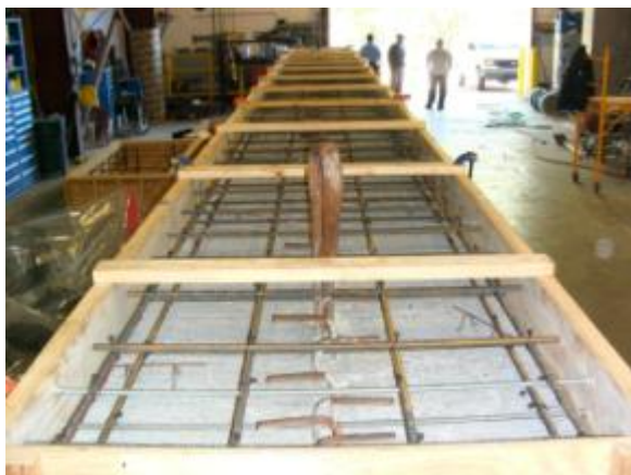
Figure 32–Deck construction A) reinforcement and B) formwork
