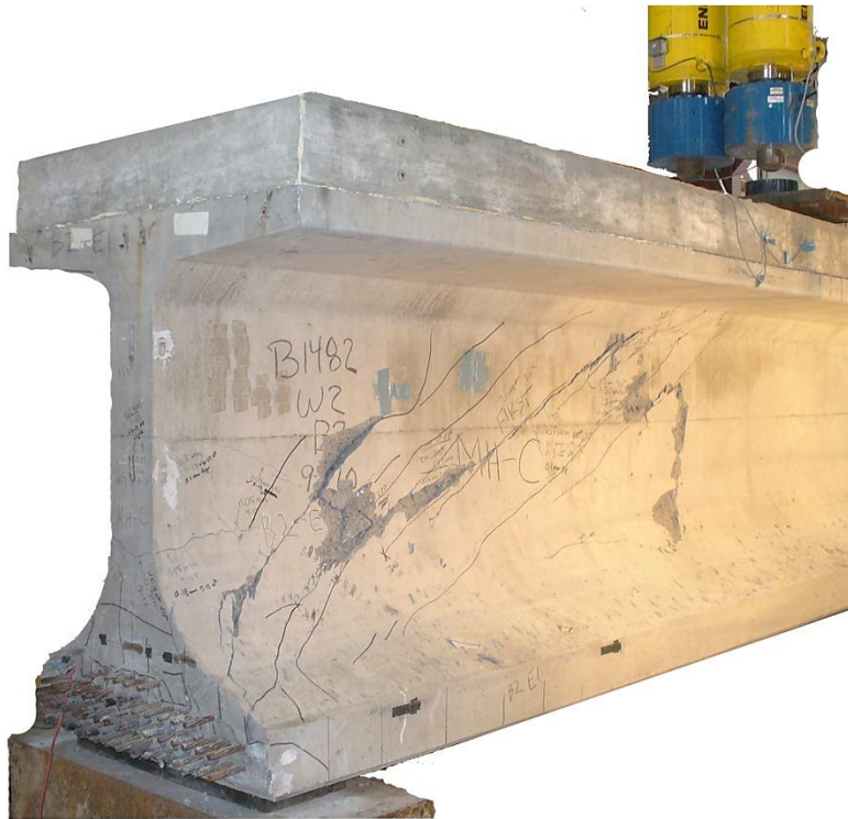
Figure 94–VC after load test
