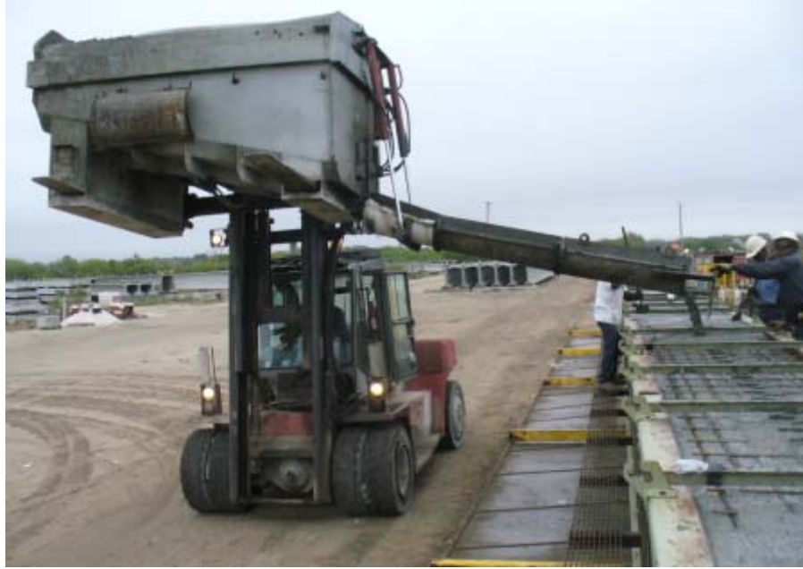
Figure 25–Concrete placement phase 2
