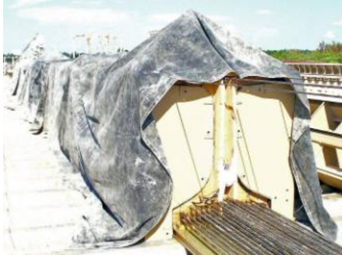
Figure 27–Girders covered with tarps
