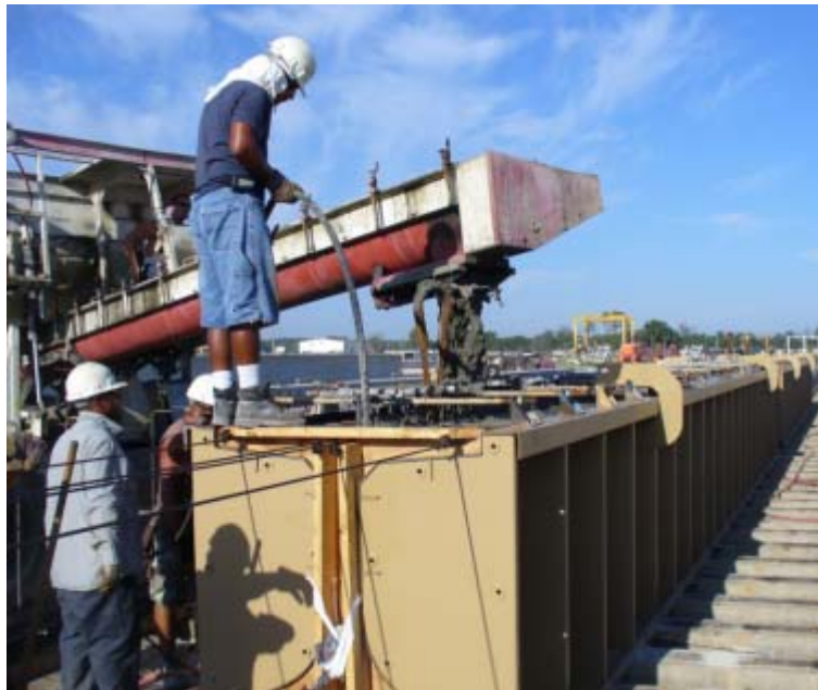
Figure 24–Concrete placement and internal consolidation phase 1
