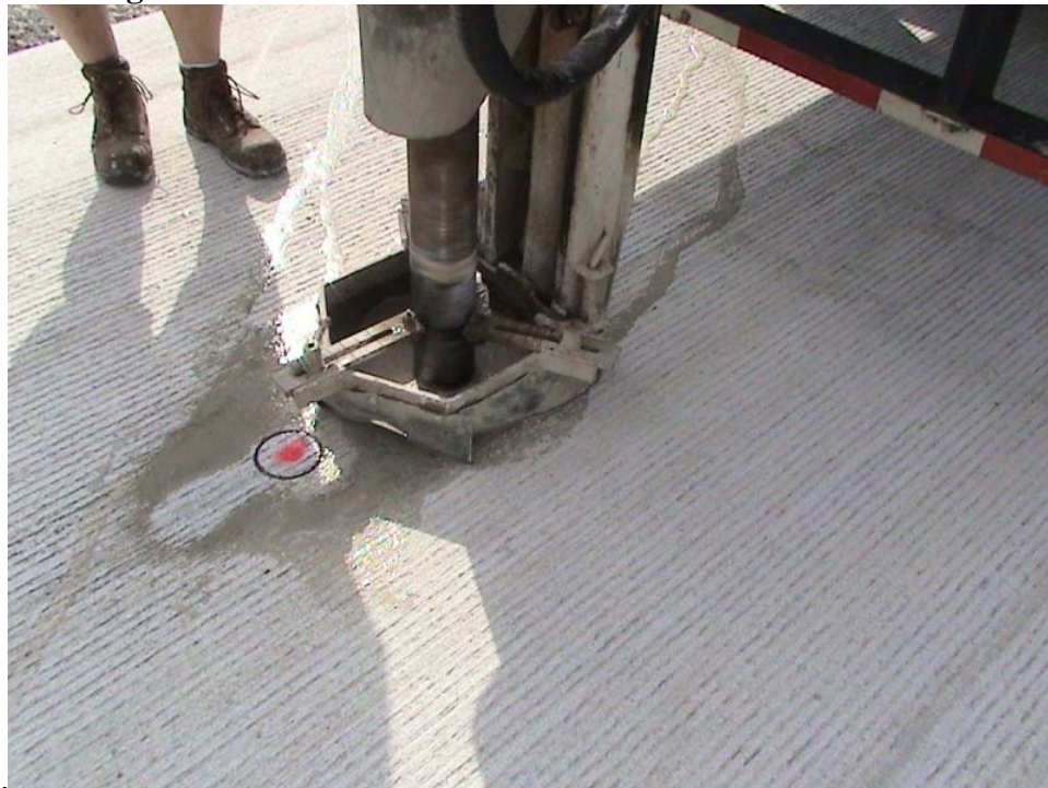
Figure 4 Coring at test locations.
