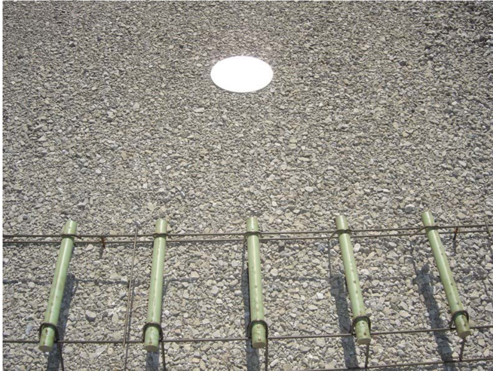
Figure 1 Target placed on granular subbase.
