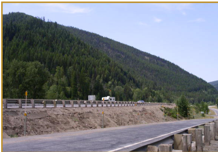
Accumulated sanding material along I 90 near Lookout Pass
