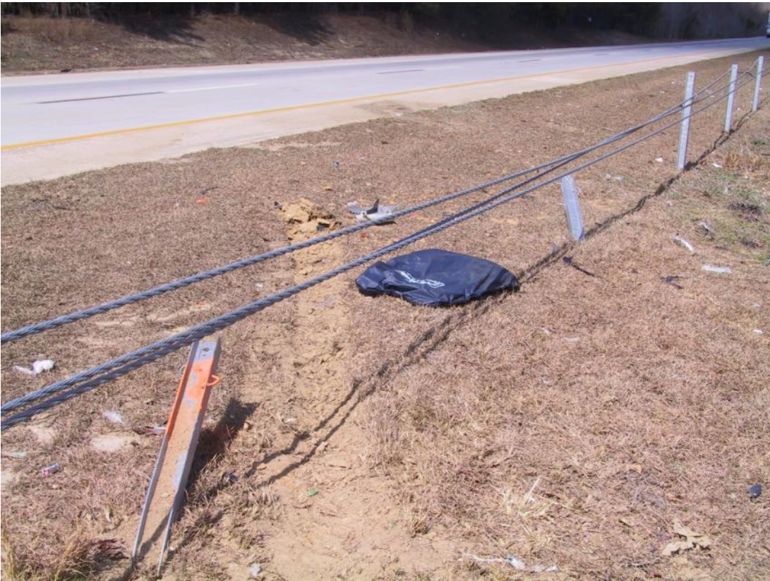
Figure 59. Diving Underride Penetration Crash in North Carolina
