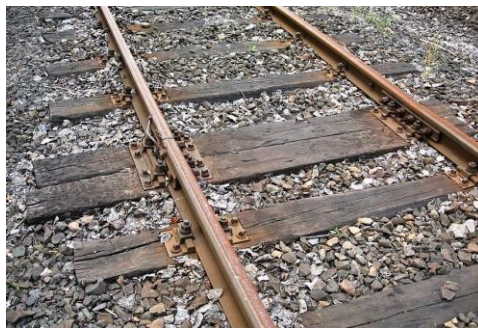
Figure 5-1: Railroad tracks on traditional wooden sleepers 40
