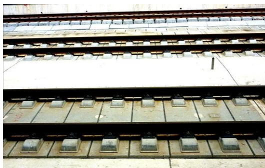
Figure 5-3: Chinese HSR ballastless tracks 42
