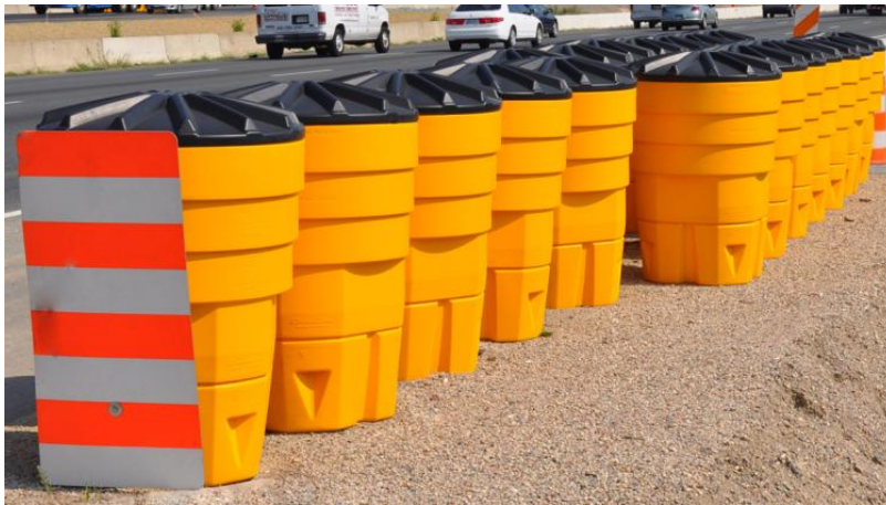
FIGURE 9 Examples of Portable Concrete Barrier End Treatments
